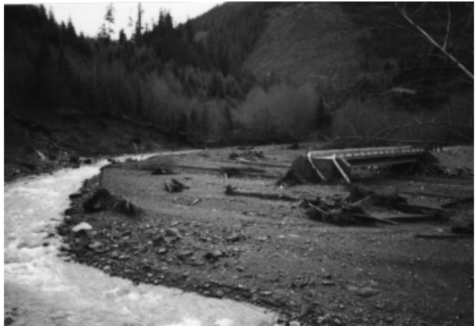
Figure 9. Canyon Creek skirts around a 100-foot bridge, removing the entire approach.
