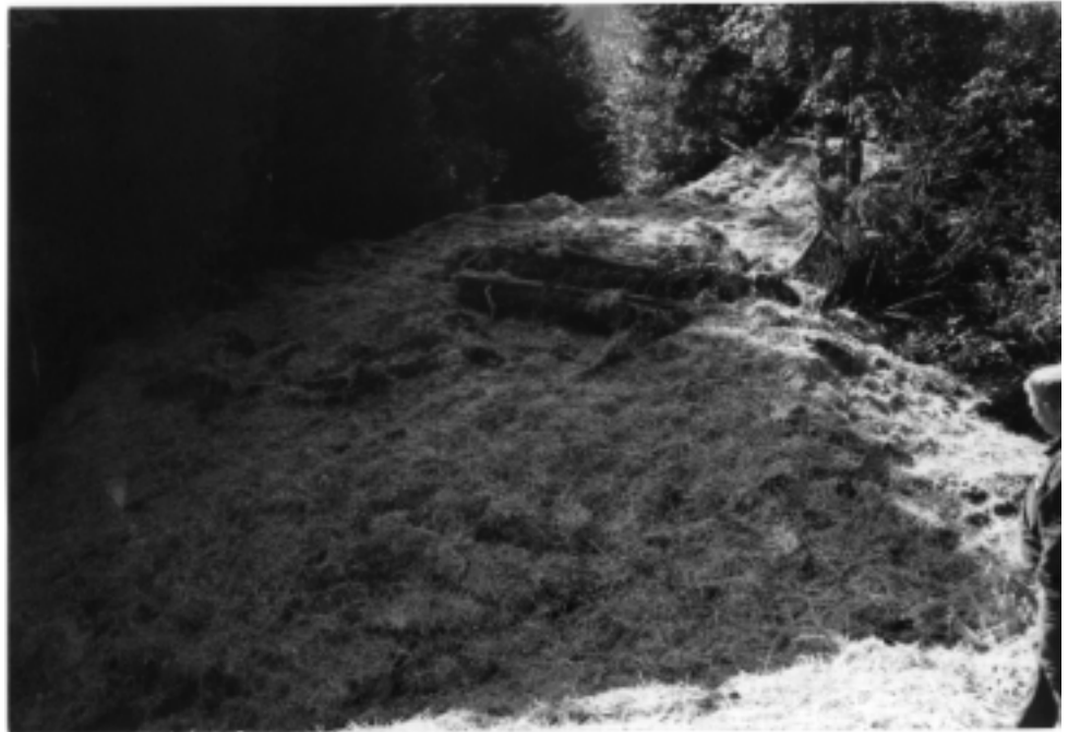
Figure 14. A decommissioned road has been seeded and mulched with straw.
