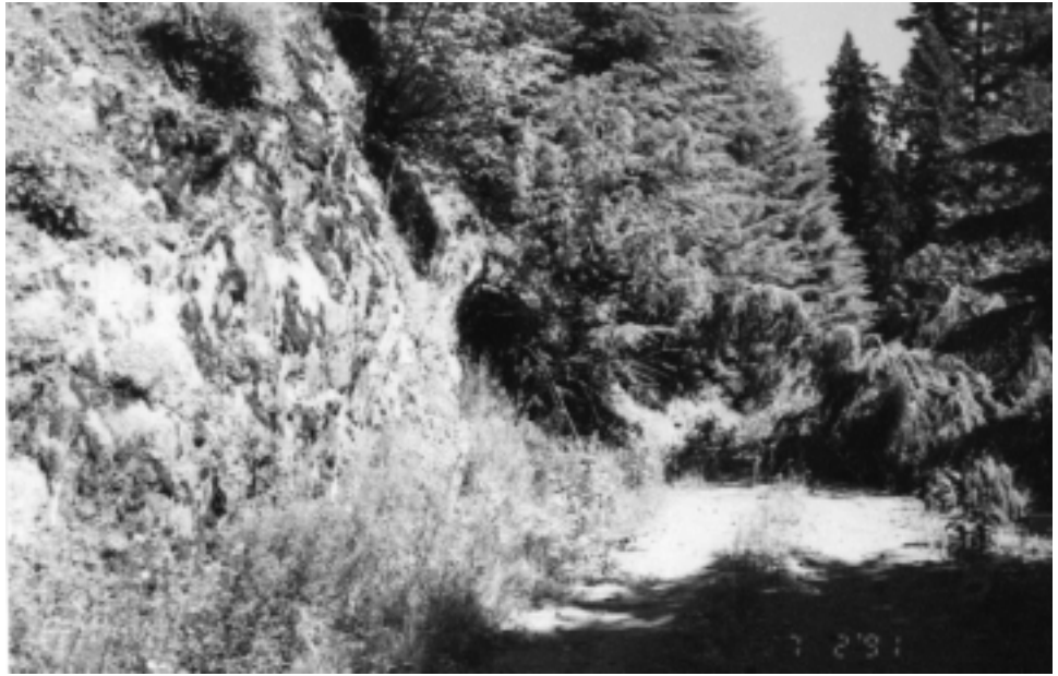
Figure 13. A low-risk road is being closed naturally by vegetation and windfalls.
