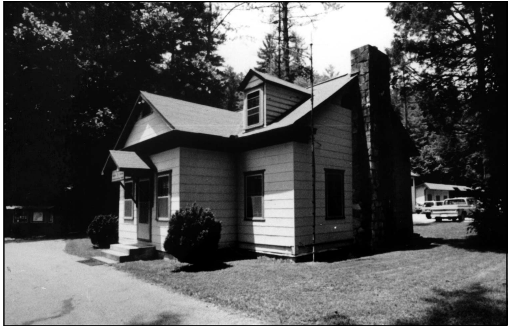
Figure 3. Older building no longer meets functional needs.
