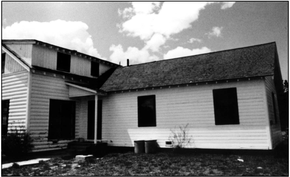
Figure 8. Bunkhouse is a combination of two buildings with an addition built in the attic. Original buildings were moved from other sites.
