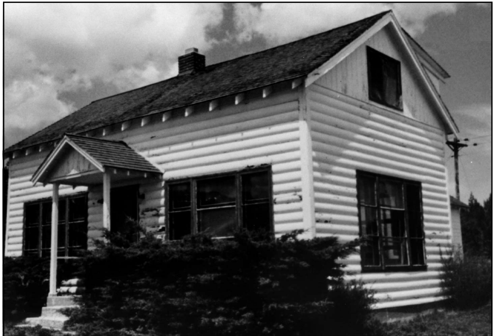
Figure 7. Bunkhouse more than 50 years old.
