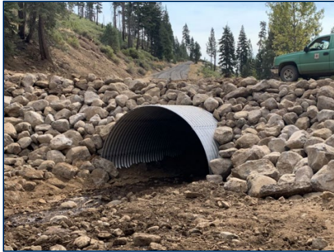
27N09 Road Hungry Creek culvert replacement.
