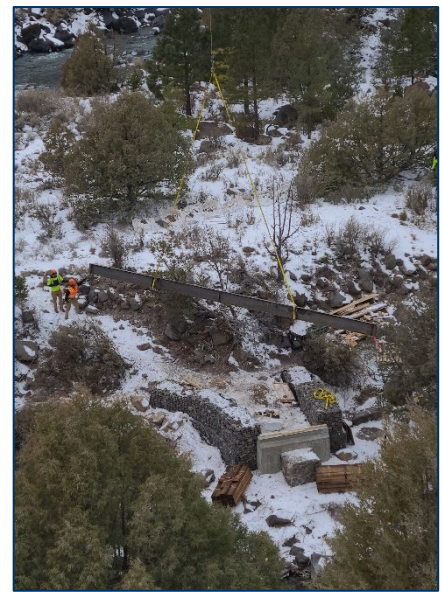
A closeup of a helicopter delivering steel beams to the site.
