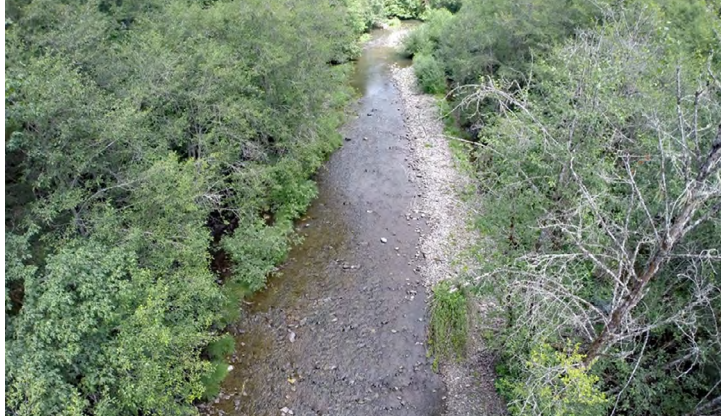
Pre-project conditions within Rock Creek; straightened stream channels and disconnected floodplains and wetland habitat. Photo courtesy of Jeff McEnroe.
