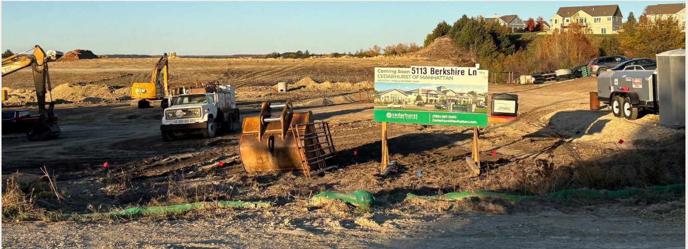
Large-scale urban development projects, such as this construction site in Manhattan, Kansas are increasingly common across the state.
