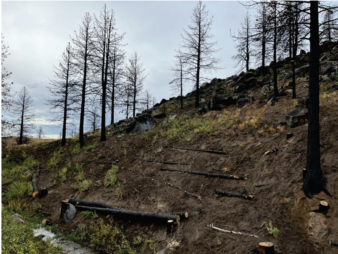
Photo 4 Log Erosion Barriers
