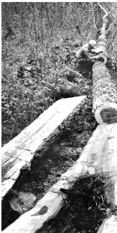
Figure 3. —Column of discoloration extending more than 30 feet above Armillaria mellea butt rot in a large sugar maple. Discoloration has joined with other discolorations entering from branch stubs, which died earlier, and now forms a nearly circular column.
