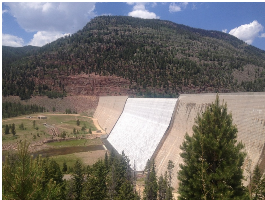
Figure 50. Upper Stillwater Dam while spilling
