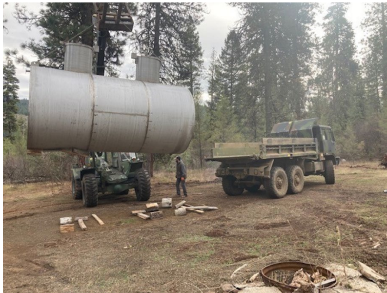
Figure 11. Installing potable water storage tank in 2022 at Third Fork Project Camp, Emmett Ranger District, 2022
