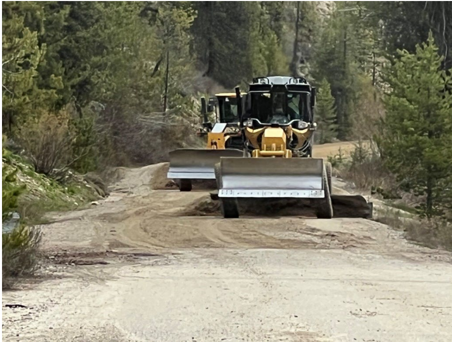
Figure 9. Road grading and aggregate placement on NFSR #698
