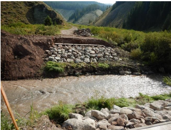
Figure 24. Bridge foundation at the TriBasin bridge project site on the Greys River. The view is looking west into the Shale Creek and East Fork Greys River drainages. Both drainages were reconnected to the Greys River through culvert removal and bridge installation. The East Fork Greys River confluence with the Greys River is upstream roughly 25 meters. Photo credit: Kelly Owens USFS, 8/24/20.
