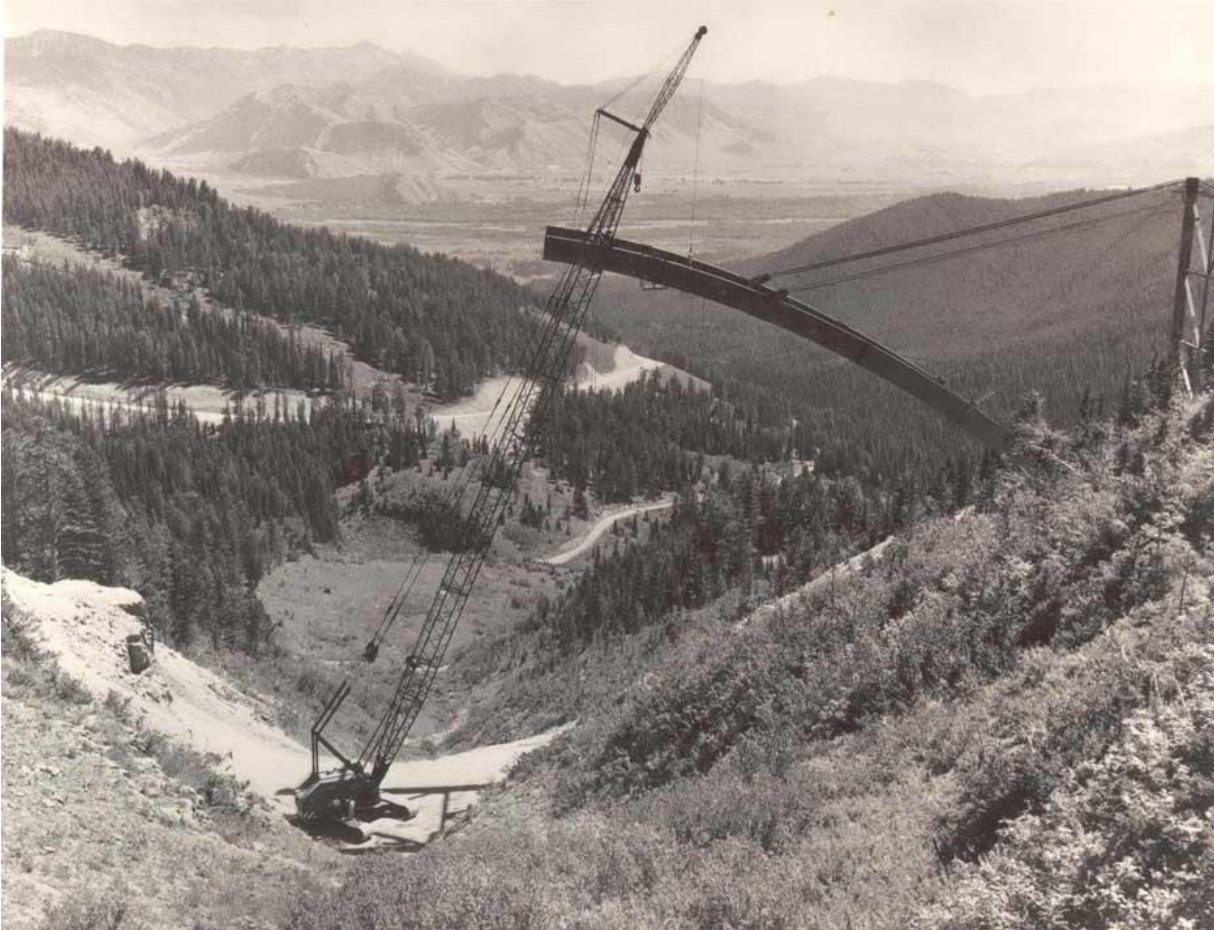
Glory Bowl suspension bridge built on new highway to shed avalanches. JHSM. bc0128.jpg.
