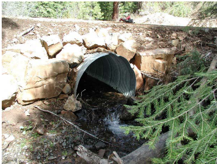
Figure 79. Culvert replaced on Stacey Creek. Photograph is looking upstream at the outlet of the culvert in the spring of 2007.
