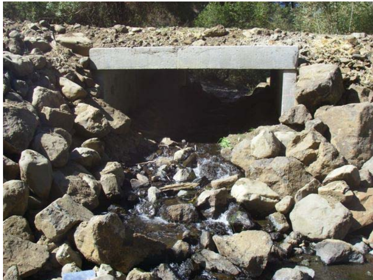
Figure 121. Bridge installed on Warm Springs Creek. Looking upstream at the outlet on September 23, 2009.
