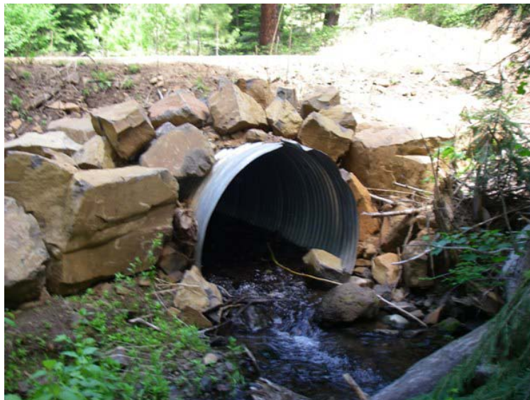
Figure 83. Culvert replaced on Stacey Creek. Photograph is looking upstream at the outlet of the culvert in the spring of 2009.
