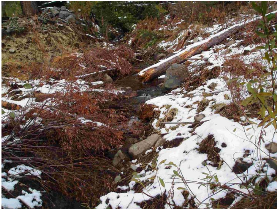
Figure 10. Tributary to Bear Creek culvert removal and channel rehabilitation.
