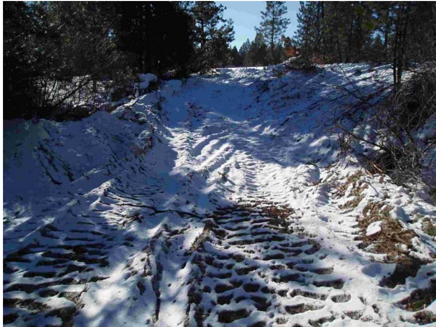
Figure 14. Snow bridge over intermittent channel at old ford in unit 12 of Bear West.
