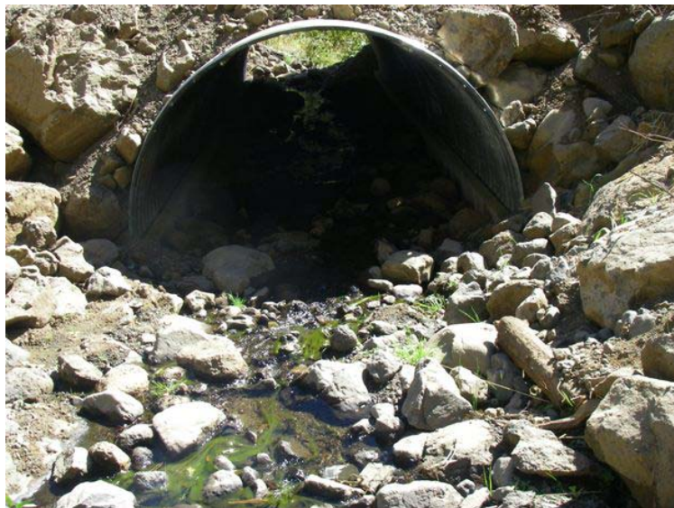
Figure 123. Culvert on Bar Creek. Looking downstream at the inlet on September 23, 2009.
