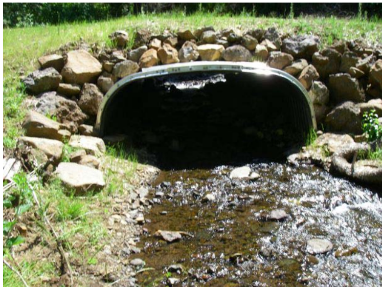
Figure 130. Open-bottom arch installed on North Grays Creek. Looking upstream at the outlet on July 15, 2009.
