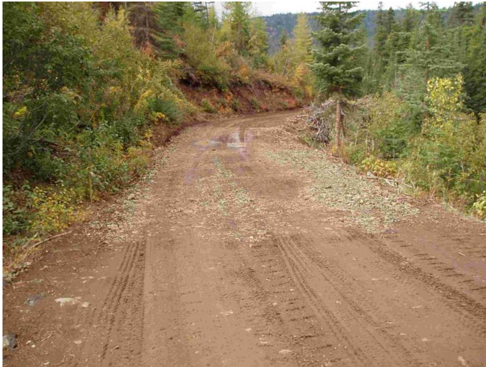
Figure 8. Road gravel mitigation implementation on Bessie Bear sale.
