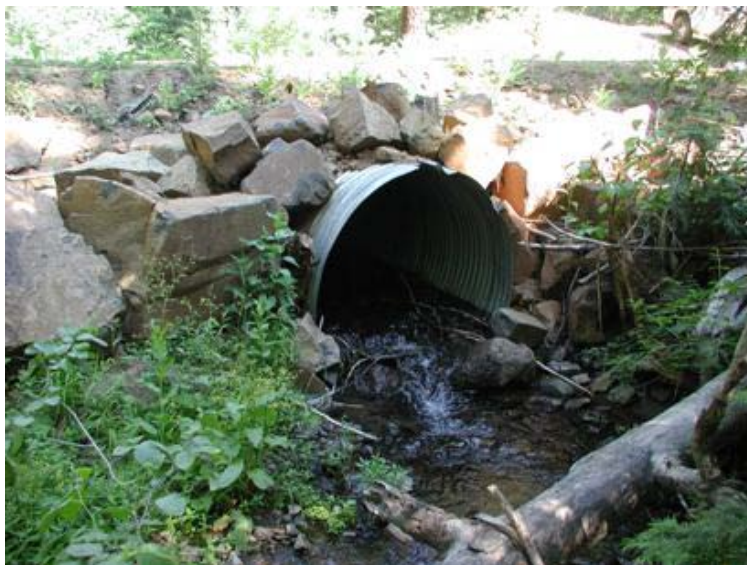
Figure 81. Culvert replaced on Stacey Creek. Photograph is looking upstream at the outlet of the culvert in the spring of 2008.
