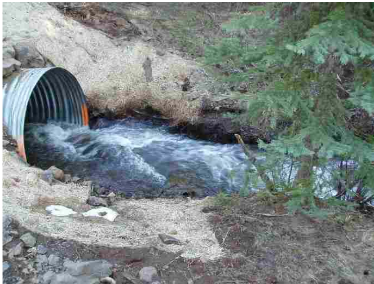
Figure 25. Inlet of the Bessie Gulch culvert on FS Road 130, May 18, 2006.
