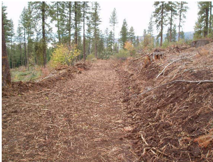
Figure 70. Temporary road within Unit 224 in the Anderson Creek Timber Sale.
