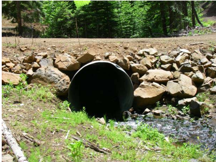
Figure 83. Culvert replaced on Stacey Creek. Photograph is looking upstream at the outlet of the culvert in the spring of 2009.
