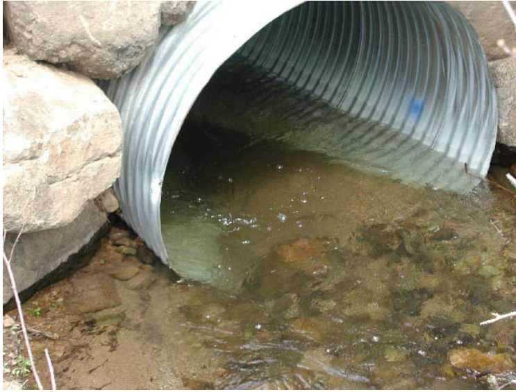
Figure 86. Culvert outlet on Fourth of July Creek. Photograph is looking at outlet pool where numerous fish were observed in 2007.
