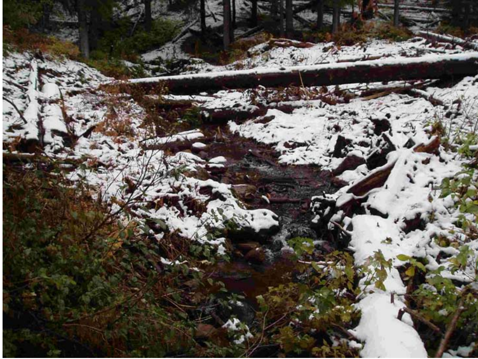
Figure 9. Wesley Creek culvert removal and channel rehabilitation.
