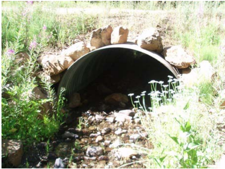
Figure 21. Outlet of the culvert on FS Road 110 (unnamed tributary of Bear Creek) on July 20, 2009.
