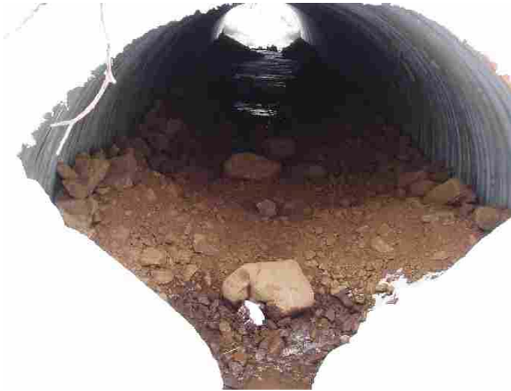
Figure 24. Outlet of the Bessie Gulch Culvert on FS Road 130, November 18, 2005.
