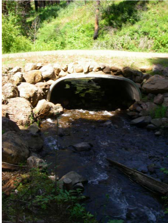
Figure 130. Open-bottom arch installed on North Grays Creek. Looking upstream at the outlet on July 15, 2009.
