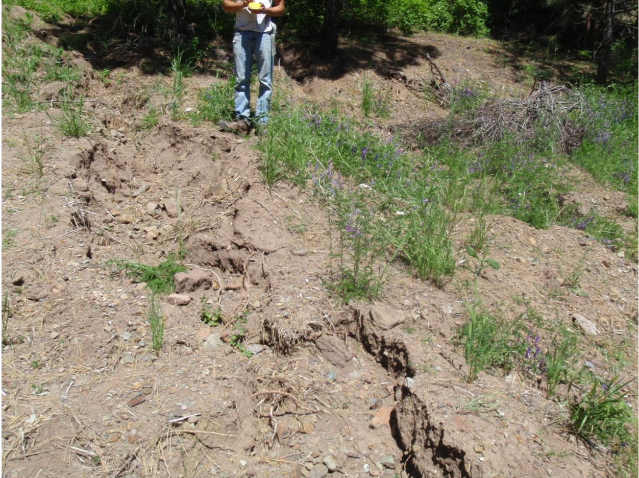
Figure 6: Gully crossing recontoured road.
