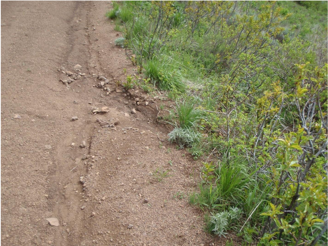
Figure 9: Non-engineered drain formed along control road.
