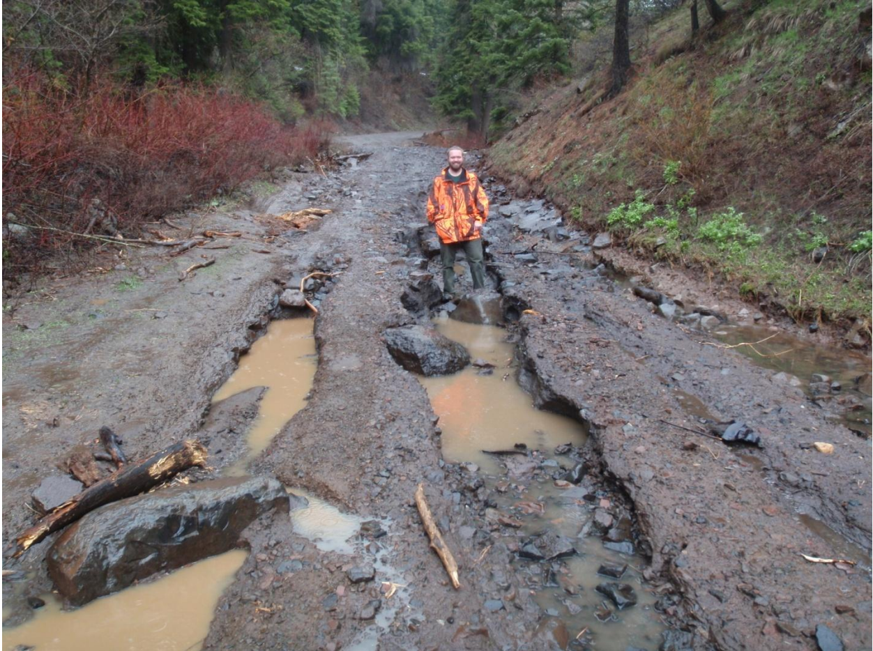
Figure 3: Damage from the April storms. The author is standing in a gullied wheeltrack where flood water was diverted down the road from the stream crossing behind the author's head.
