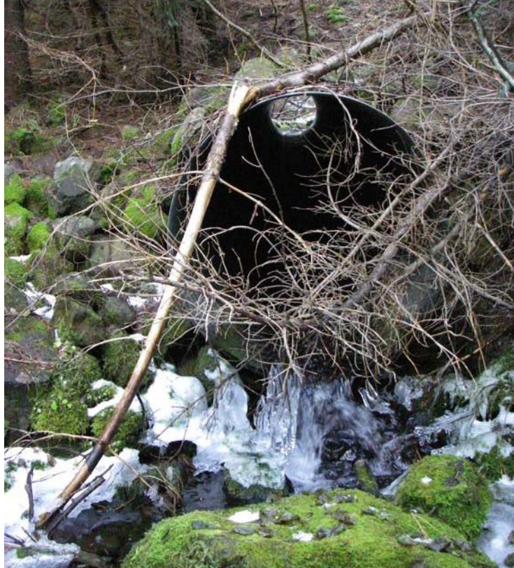
Figure 6. Upper culvert encountered on Cold Springs Creek on November 05, 2009. Culvert is a potential fish passage barrier. Fish were not captured at the electrofishing site immediately upstream of this culvert.
