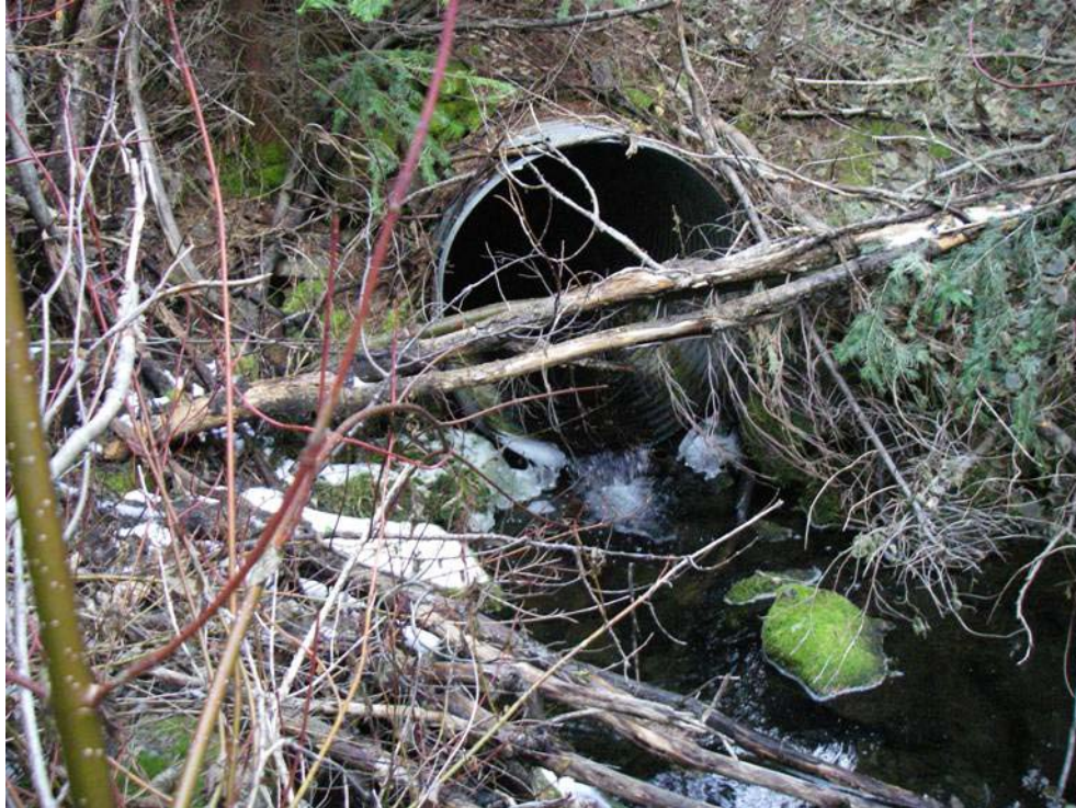
Figure 6. Upper culvert encountered on Cold Springs Creek on November 05, 2009. Culvert is a potential fish passage barrier. Fish were not captured at the electrofishing site immediately upstream of this culvert.
