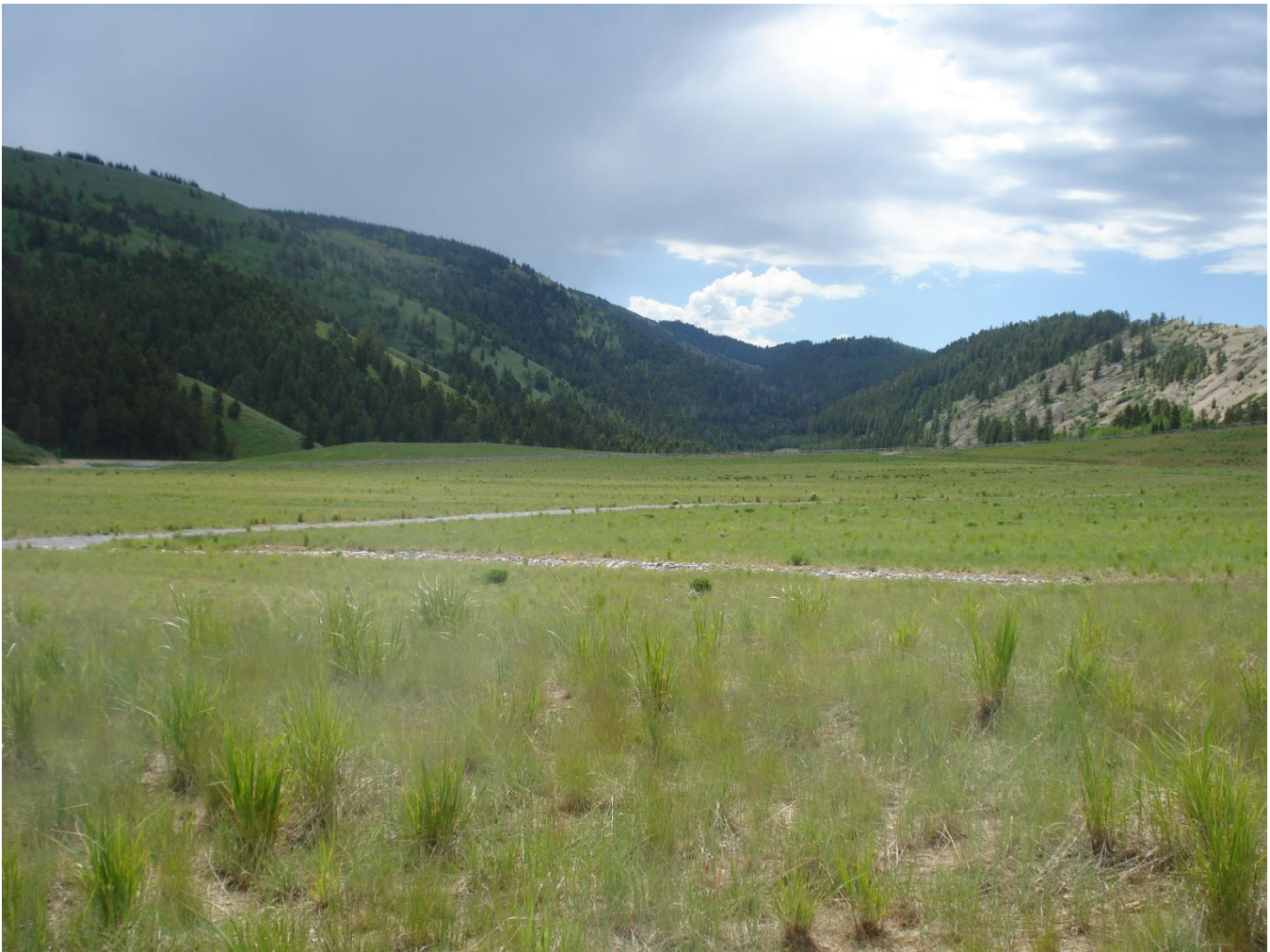
Picture 17 (facing southeast): Picture of the top deck of SMCM CVF with vegetation growing and drainage features. Various grasses were observed with some sagebrush growing.
