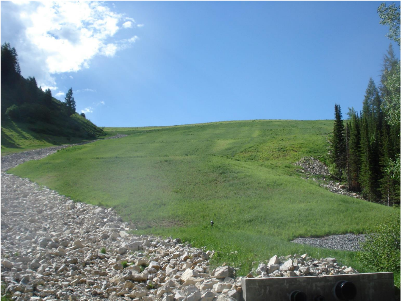
Picture 4 (facing southeast): Toe of SMCM CVF pointed up the face of the revegetated cap and cover.
