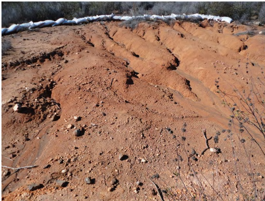
Photograph A-6: View northwest of headwall of erosion scarp and rutting from surface water flow downslope towards burn dump. Engineering Evaluation/Cost Analysis, Cleveland National Forest, Ramona, California
