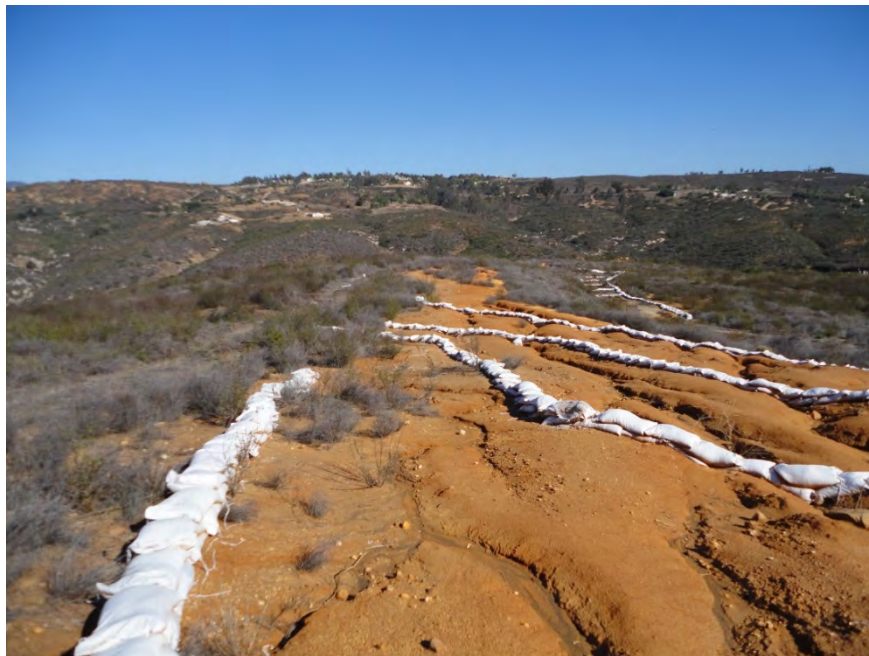
Photograph A-4: View east of berm at the north boundary of the Ramona Burn Dump and sandbags and erosion rutting. Engineering Evaluation/Cost Analysis, Cleveland National Forest, Ramona, California
