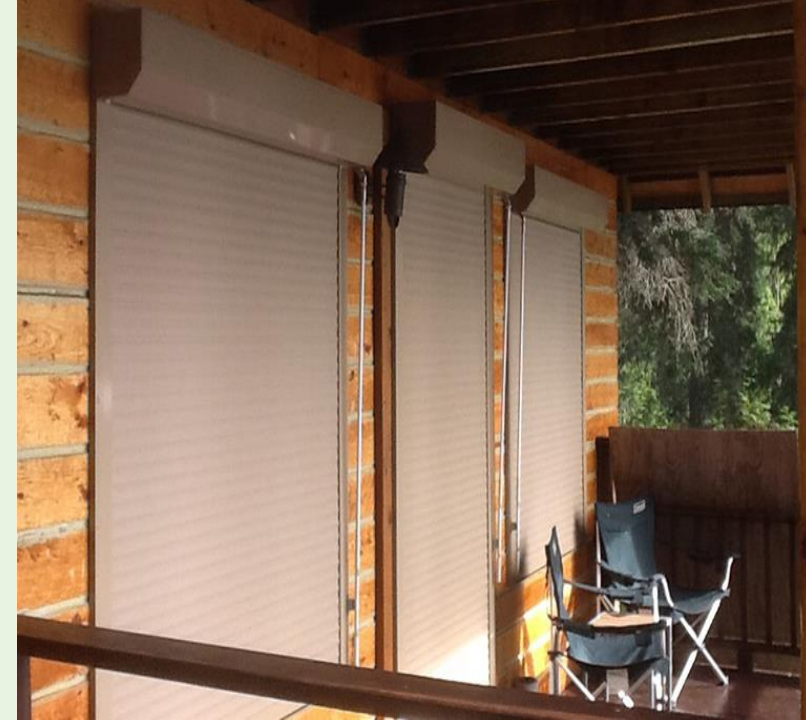
Rolling steel shutters
