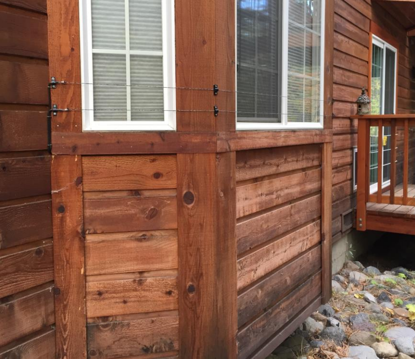
Electric fencing along windows
