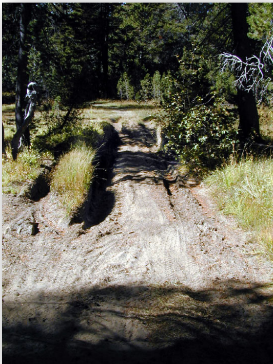
Many non-system routes lack water drainage which can cause damage to the road, adjacent vegetation, and other resources.
