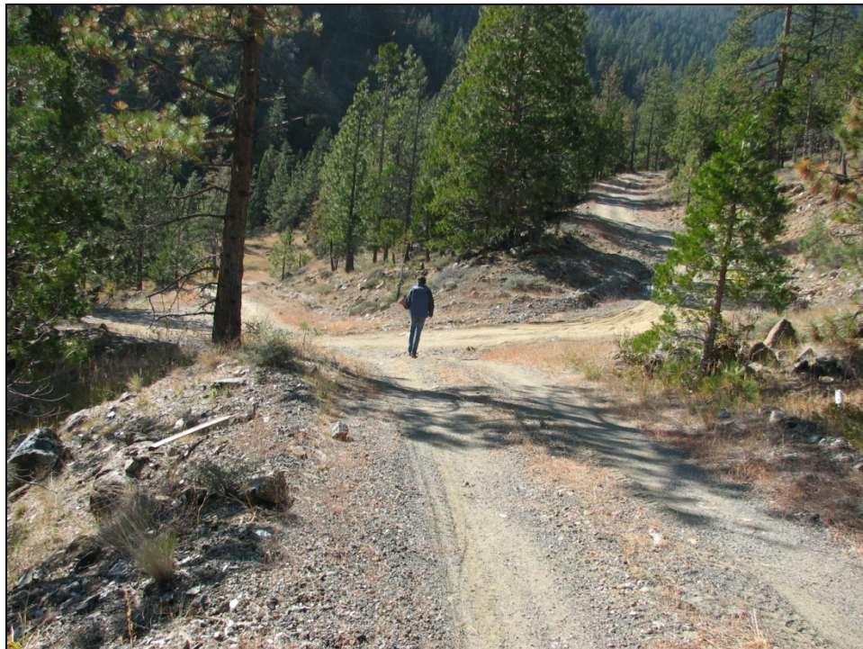
PHOTO 3-29: ROAD 42N19- MANY SWITCHBACKS MAKE IT DIFFICULT TO CONTROL ROAD RUNOFF.
