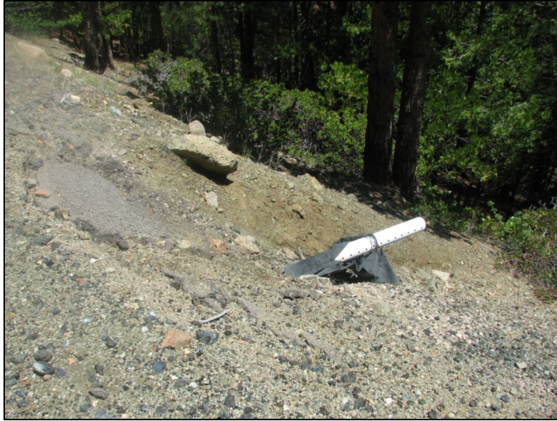
PHOTO 3-23: PARKS CREEK ROAD 42N17- PERFORATED PIPE BELOW ROAD (EARLIER ATTEMPT AT DEALING WITH SUBSURFACE WATER) WHERE FILL IS SETTLING.
