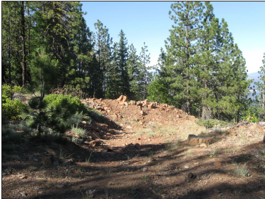
PHOTO 3-17: A FUNCTIONING ROAD CLOSURE BERM (NORTH STATE RESOURCES 2010).
