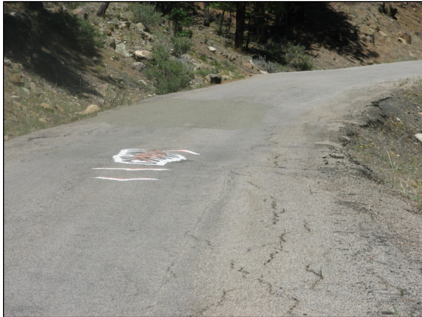
PHOTO 3-22: PARKS CREEK ROAD 42N17- SETTling OF FILL AND BUCKLING OF PAVEMENT NEAR STEWART SPRINGS.
