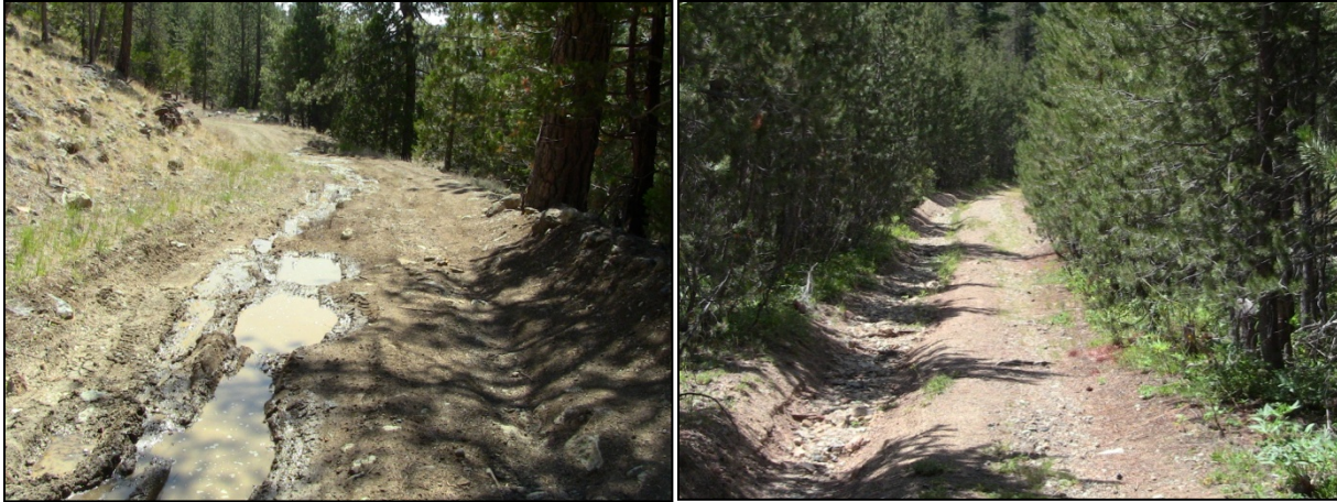
PHOTO 3-34 AND 3-35: DRAINAGE ISSUES ON ROADS 42N19 (LEFT) AND 41N74 (CALDWELL LAKES ACCESS).
