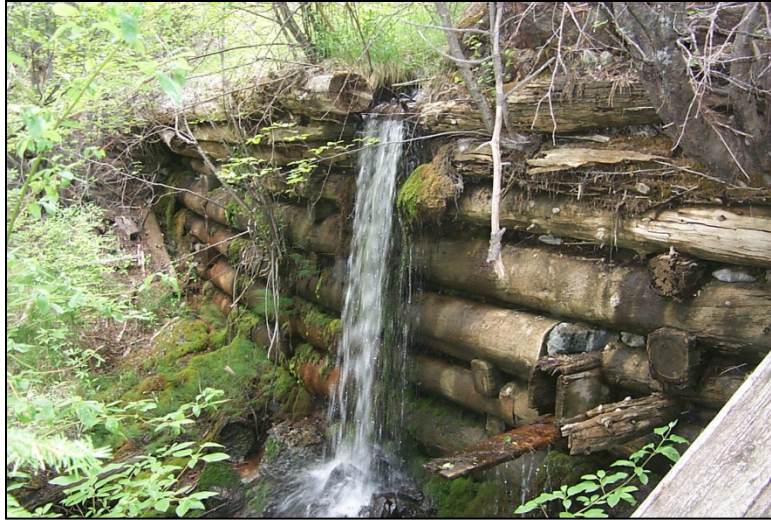
PHOTO 3-37: OLD LOG DAM ON SOUTH FORK WILLOW CREEK ASSOCIATED WITH HISTORIC MINING OPERATIONS, 2001.
