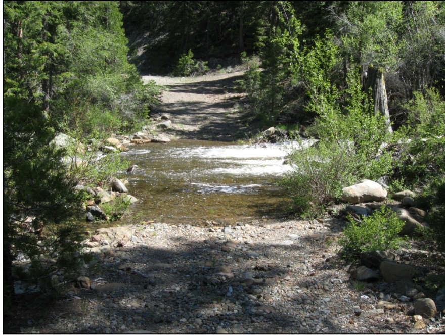
PHOTO 3-14: A FORD WATER CROSSING (NORTH STATE RESOURCES 2010).
