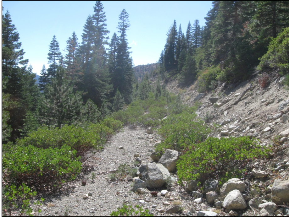
PHOTO 1-16: SLIDE MATERIAL AND VEGETATION HAVE CLOSED THIS ROAD (NORTH STATE RESOURCES 2010).
