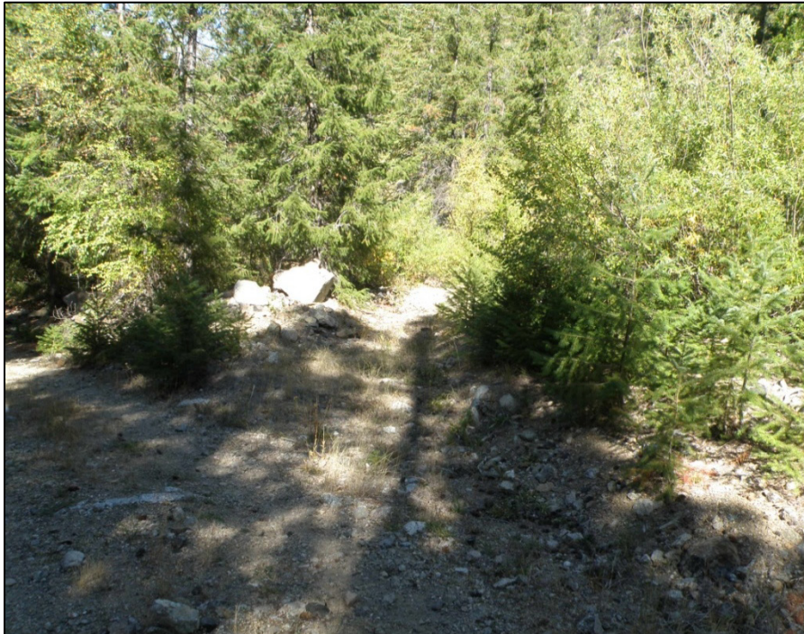
PHOTO 3-40: ROLLING DIP ON DEWEY MINE ROAD, UPSTREAM FROM THE MAIN CYANIDE PROCESSING PLANT.
