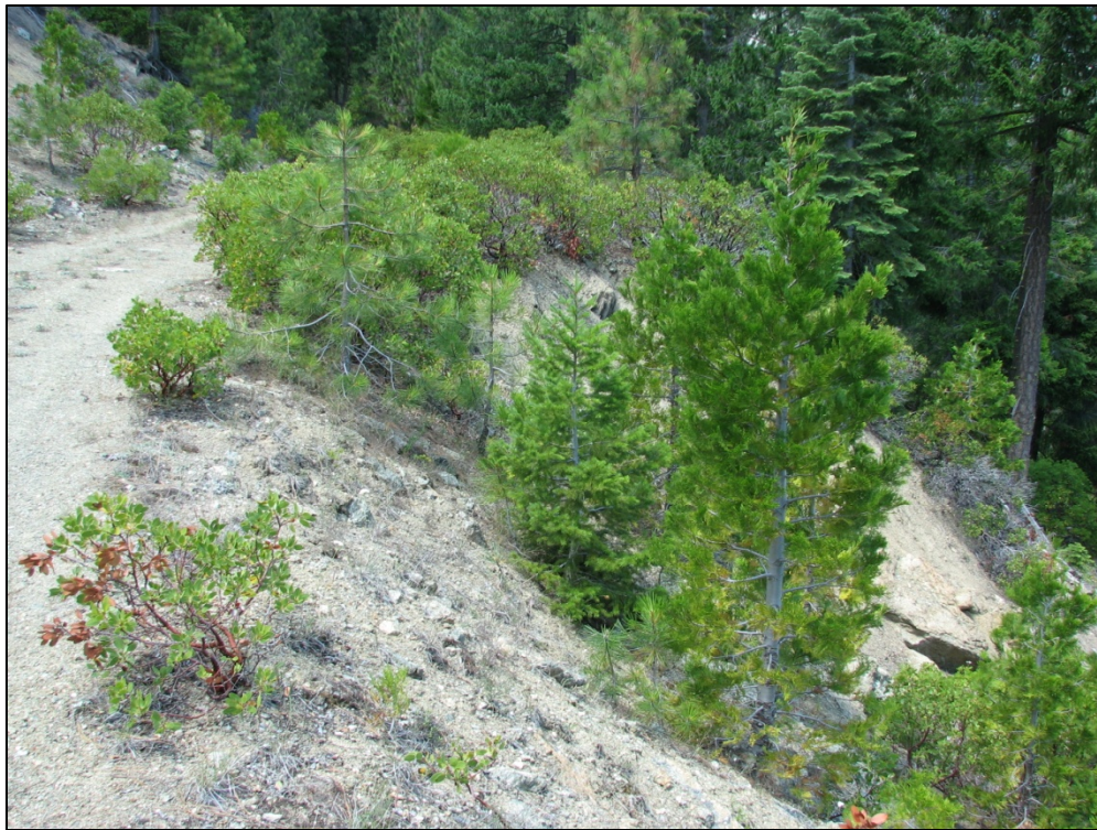
PHOTO 3-24: FILL FAILURE ABOUT 20 YEARS OLD ALONG ROAD 41N16Y.
