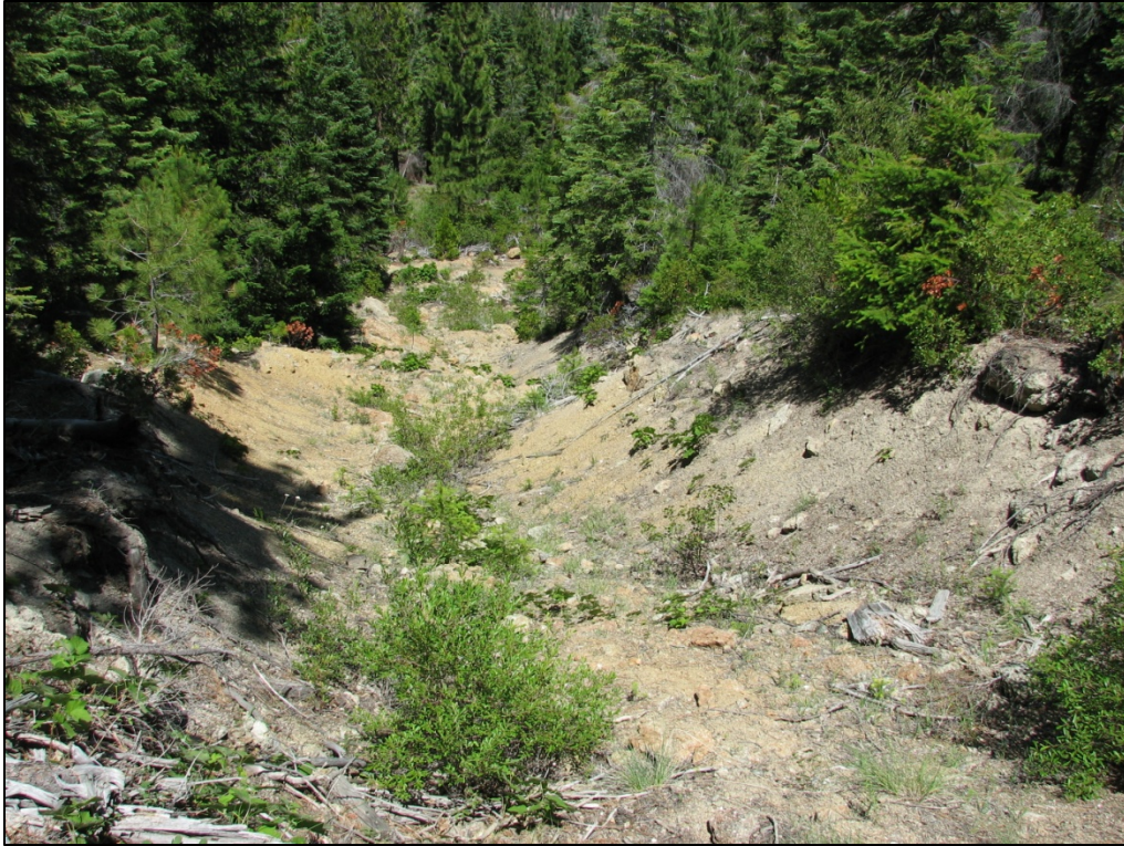
PHOTO 3-27: LANDSLIDE ABOVE ROAD 41N16Y- VIEW DOWNHILL, DEBRIS COVERS THE ROAD AT THE BOTTOM OF PHOTO.
