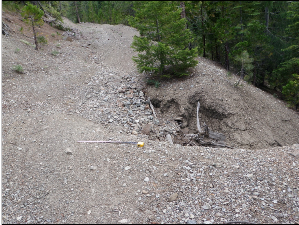
PHOTO 3-15: A LACK OF MAINTENANCE AND EROSION CONTROL CREATES POOR ROAD CONDITIONS AND SAFETY CONCERNS (NORTH STATE RESOURCES 2010).
