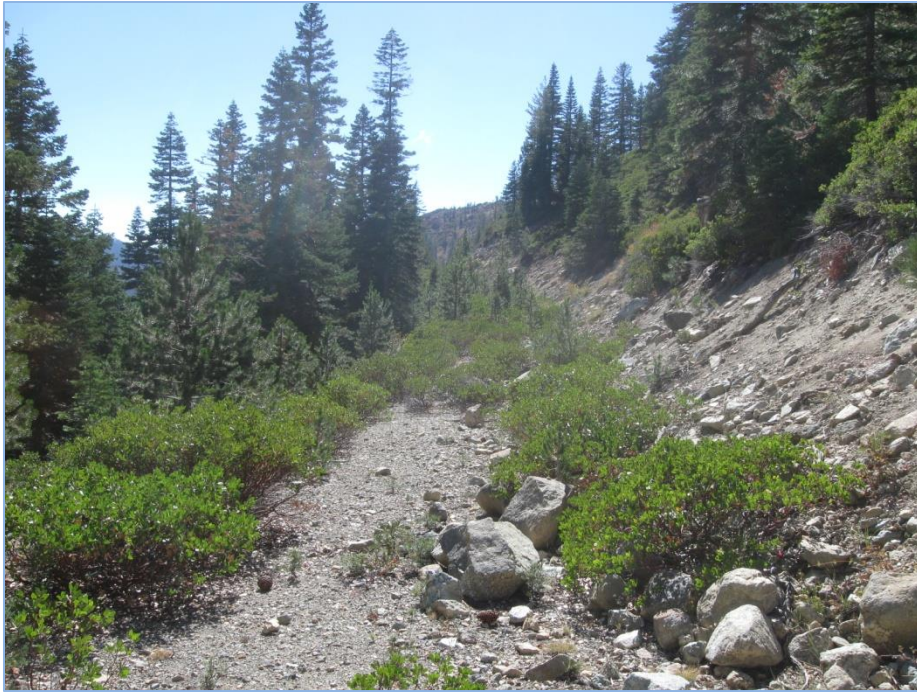
Figure 4. Slide material and vegetation have closed this road (North State Resources 2010)
