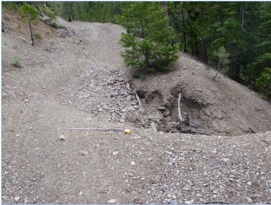
Figure 3. A lack of maintenance and erosion control creates poor road conditions and safety concerns (North State Resources 2010)
