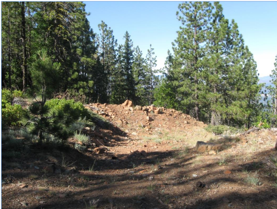
Figure 5. A functioning road closure berm (North State Resources 2010)
