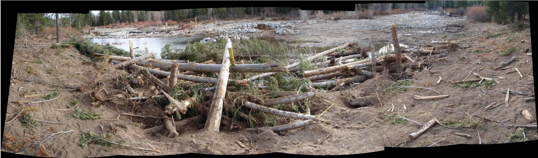
PP 18A Panorama 11/09/2009 Post Construction.
