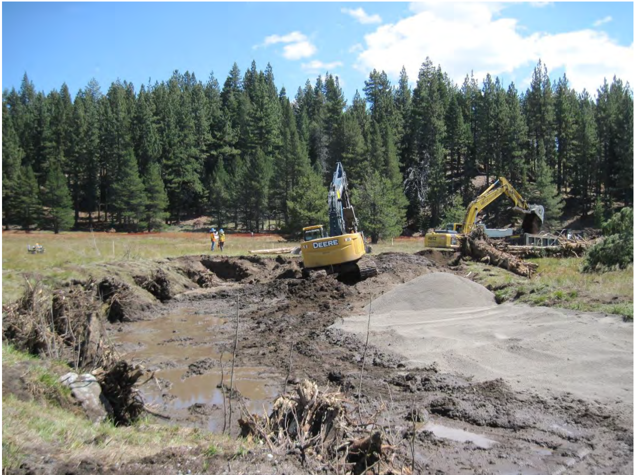
Photos of rootwad revetment pool bank treatment during construction and 2 years post-project
