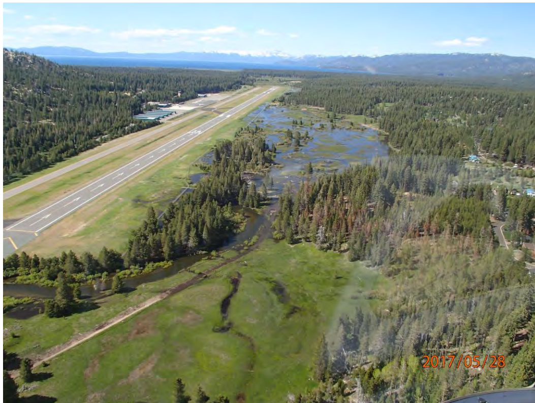
Aerial photos of Reach 5 project area from 5/28/2017, approximate 775 cfs flow
