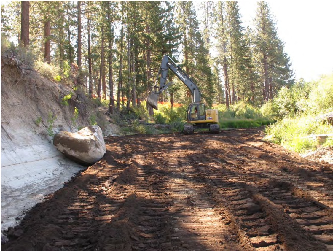
Photos of northern inset floodplain and former channel backfill during construction and 2 years post-project
