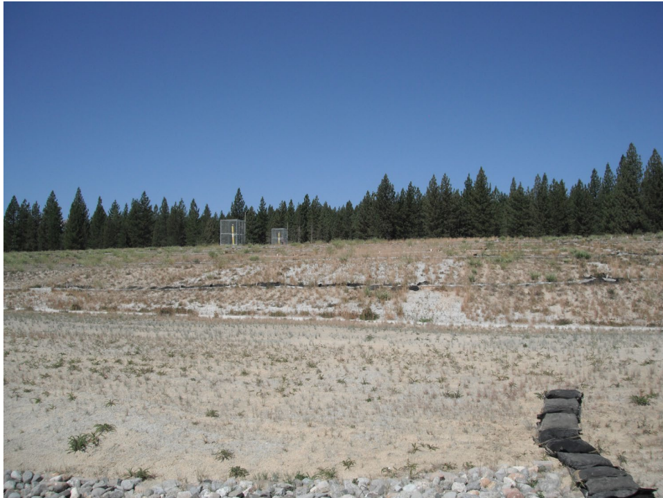
Meyers Landfill Cap and Gas Vents Photo 2014
