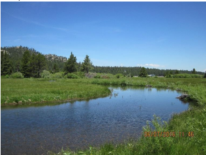
Completed Reach 5 channel
