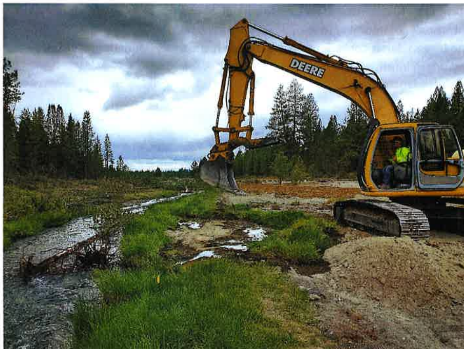
Figure 1. Mulch and slash placement to address sedimentation along Paulina Creek
