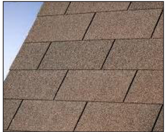
Composition shingles—acceptable
