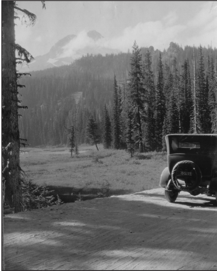
The Mt. Hood Loop Highway, ca. 1925.
