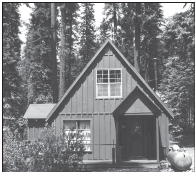
Example of small Rustic style cabin
