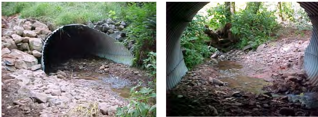
Figure 28 Two views of the same culvert. Notice the culvert is large enough to accommodate high water flows. The rocks on the bottom recreate natural stream flows, which allow passage of aquatic organisms through the pipe.
