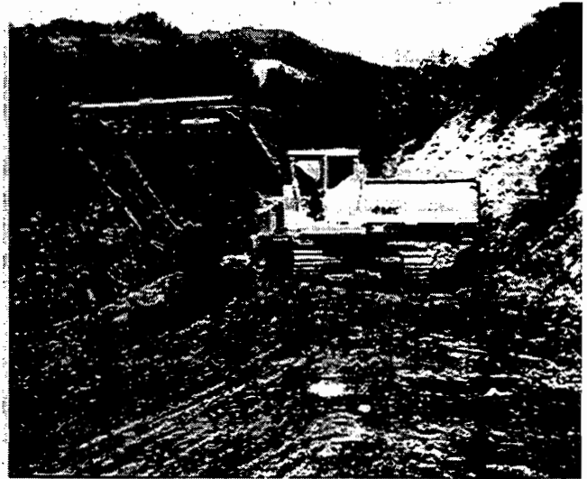
Figure 14. A track mounted excavator retrieves unstable material slopes from early sidecast road construction in the mid 1980's.
