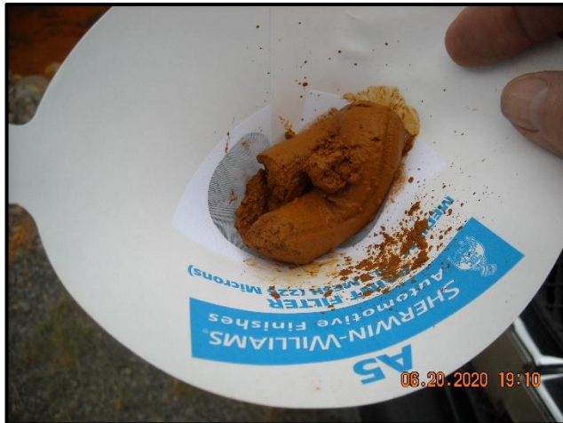
Photo 13. Successful paint filter test (No water!)
