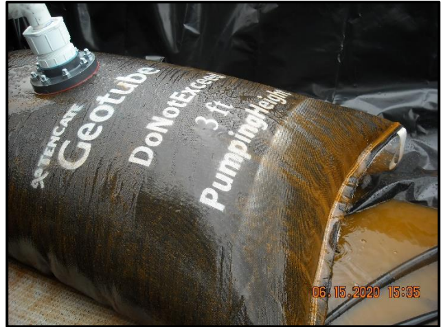
Photo 8. Active Geotube filtering
