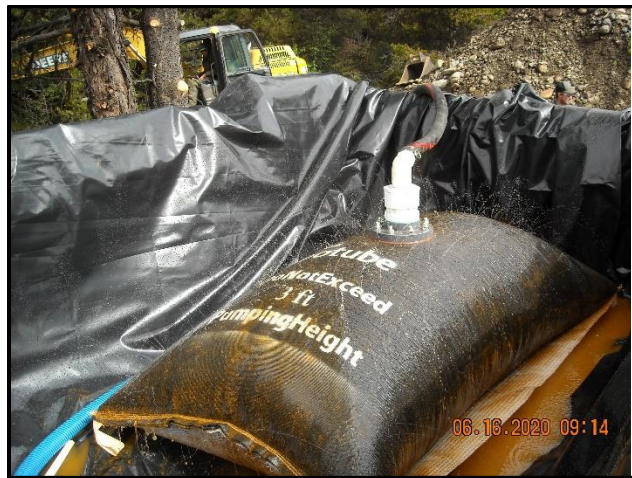
Photo 9. Geotube filtering at high pressure
