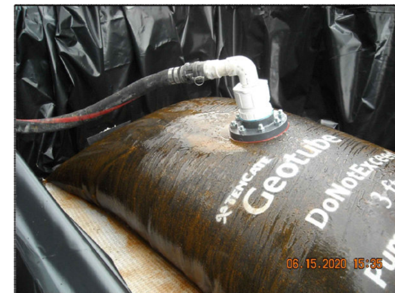
GEOTUBE IN DUMP TRUCK AT BLUEBIRD SETTLING PONDS DURING PUMPING OPERATIONS
