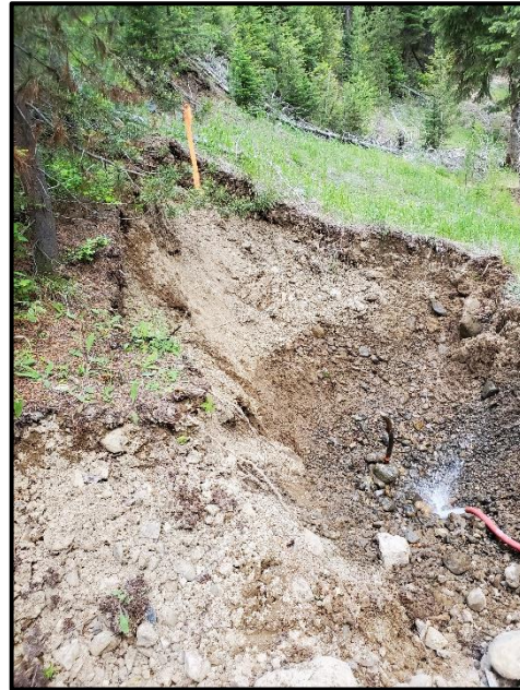
Photo 19. Infiltration test, BLK-TP2
