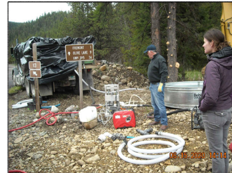
PUMPING OPERATIONS AND POLYMER MIXING AT BLUEBIRD SETTLING POND
