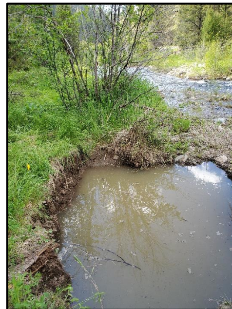
Photo 21. Pit exposing pipeline
