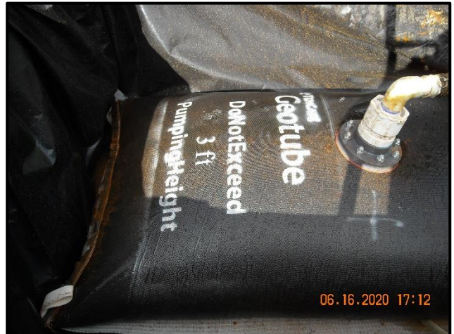
Photo 12. Active filtering at Blackjack Pond
