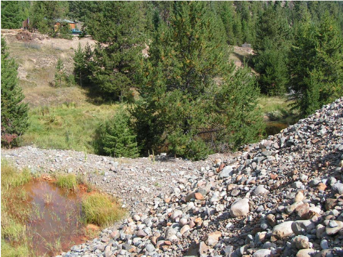
North end of Bluebird settling pond adjacent to private property (note seepage on other side).
