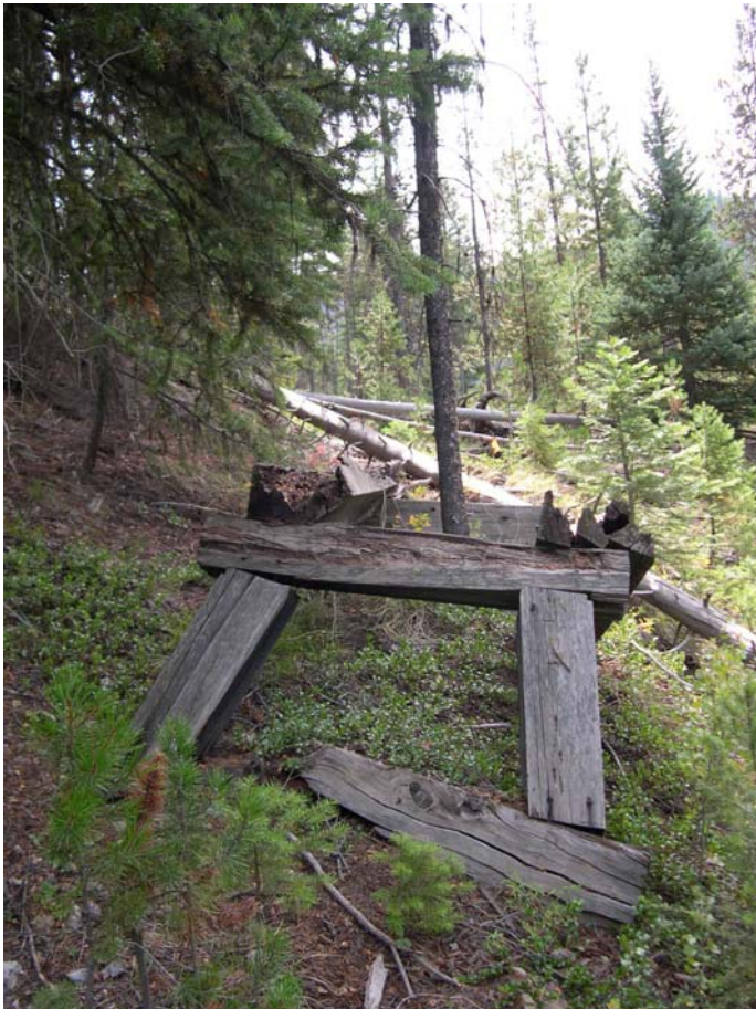
East of north waste rock pile showing end of track supports.
