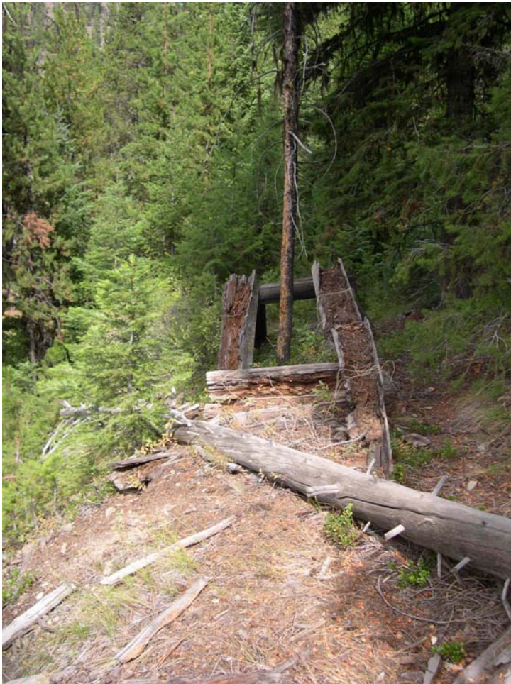
View of north waste rock pile showing remains of timber track supports.
