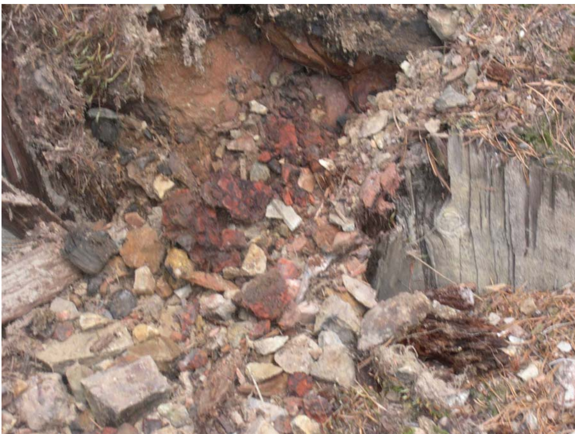
Outside edge of burned mill site structure.
