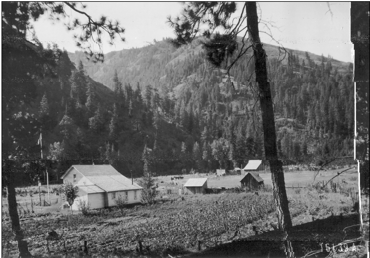
Plate 1: “Tucañon Ranger Station” (photograph taken by M.N. Unser in 1913). According to a history of the northern Blue Mountains by Gerald J. Tucker (1940), this ranger station cabin was constructed in the fall of 1907. The structure was rehabilitated by the Forest Service in the early 2000s (with much of the work occurring in 2002). It is interesting that this structure was originally built by a contractor (rather than the Forest Service), and it is the oldest contractor-built Forest Service structure in the Pacific Northwest Region.
