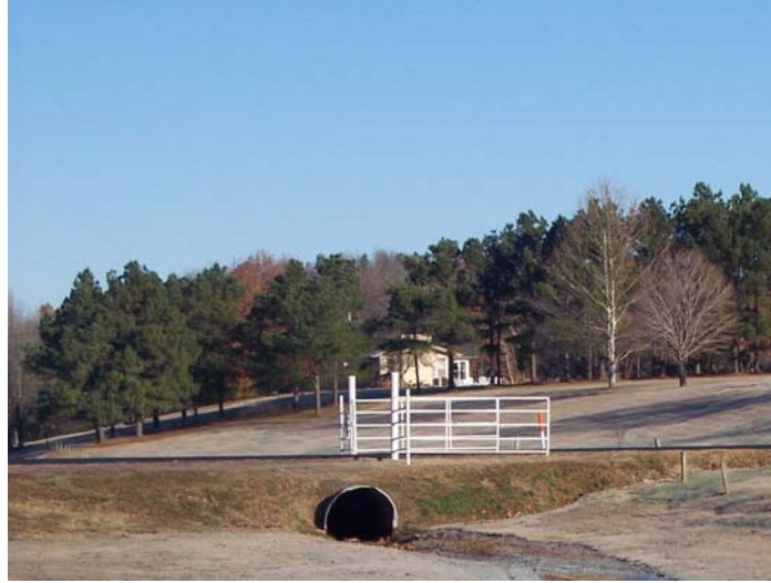
Downstream side of the culvert with barrier removed and channel restored.
