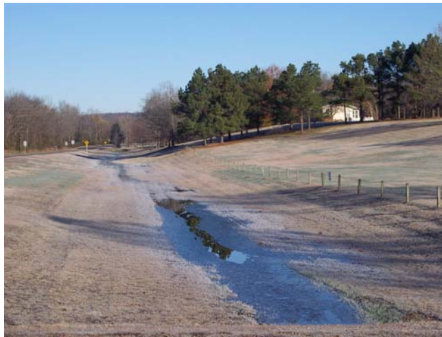
Upstream side of the culvert with restored channel instead of pooled habitat.
