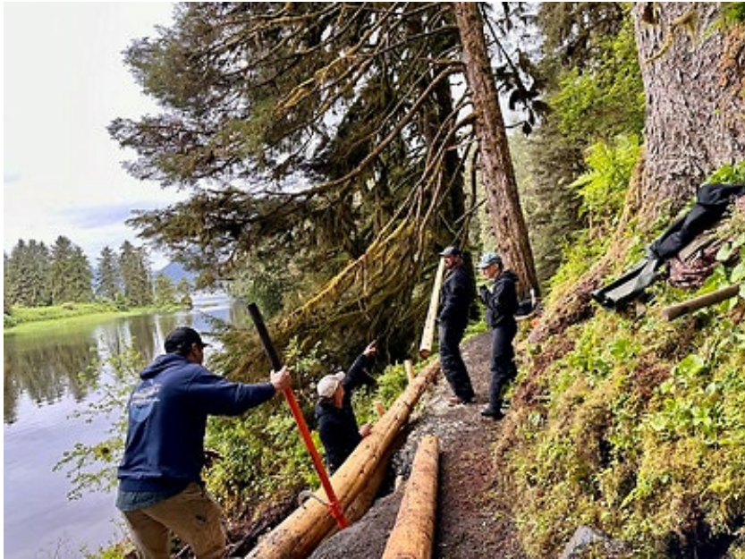
Figure 5. Wrangell Ranger District trail crew repairs a trail after winter blowdown and erosion. USDA Forest Service photo by Jennifer Kardiak.
