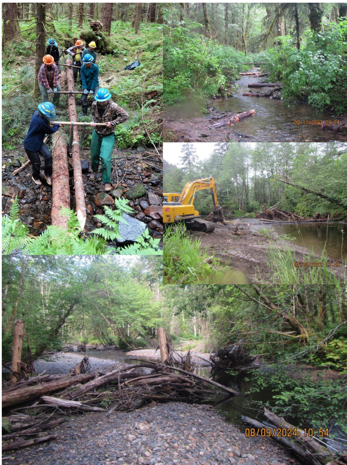
Figure 12. Photo collage of aquatic habitat improvement projects. Upper left: hand crew working on stream restoration in Sprout Creek of the Margaret Creek priority watershed. Upper right: completed hand crew stream restoration in Last Chance Creek. Middle right: excavator working on stream restoration in the Margaret Creek priority watershed. Bottom: completed stream restoration work in the Margaret Creek priority watershed. Photo credit Jonathan Hyde.
