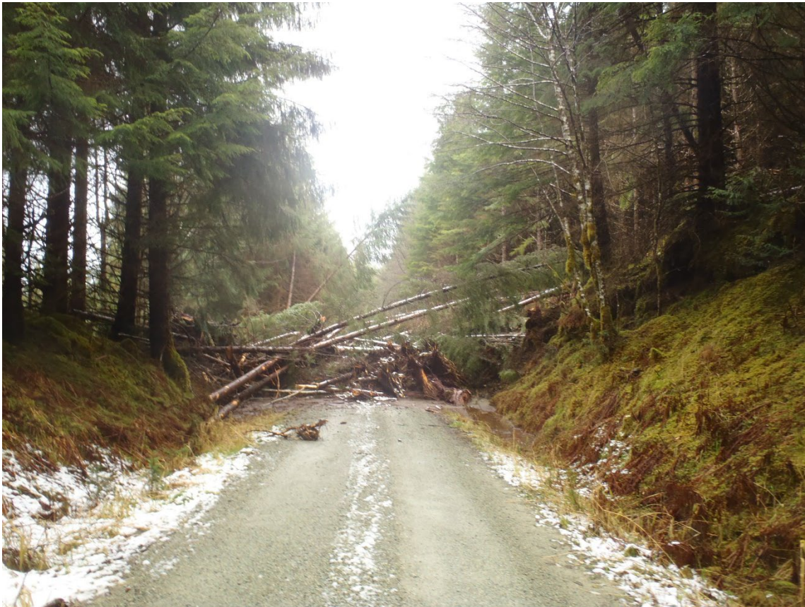
Figure 5. A small landslide that deposited debris on a gravel road, showing an example of an impact of geologic hazards to infrastructure.
