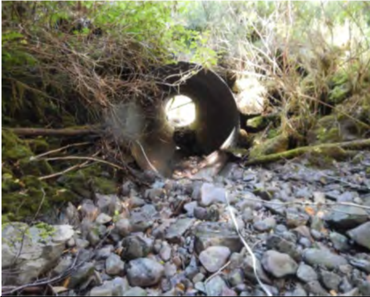
2050000 MP10.36 Outlet looking upstream.
