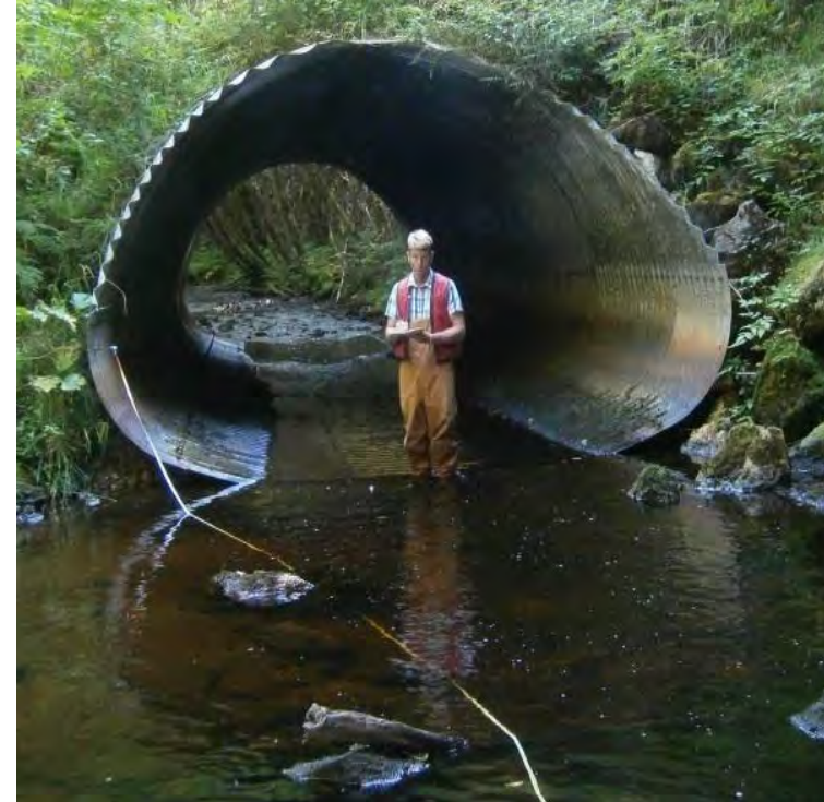
2051000 MP1.42. Outlet looking upstream.
