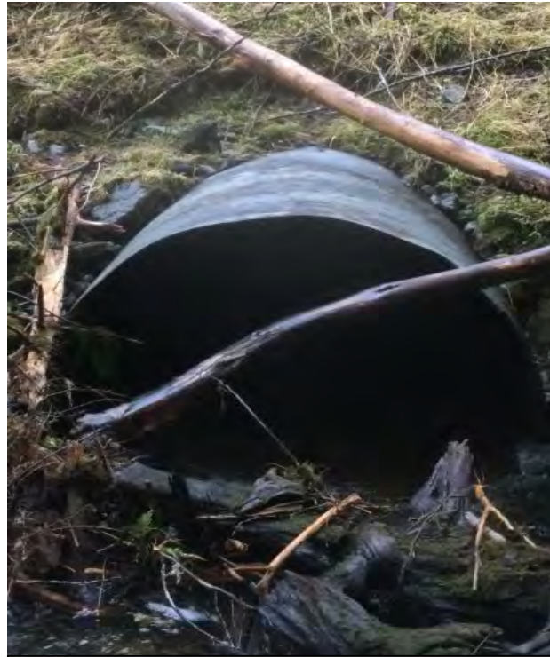
2050000 MP19.51 Outlet looking upstream.
