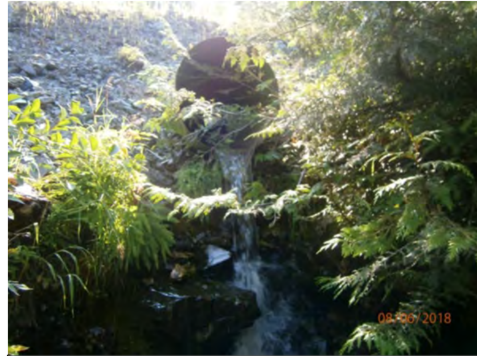
2050000 MP14.69 Outlet looking upstream
