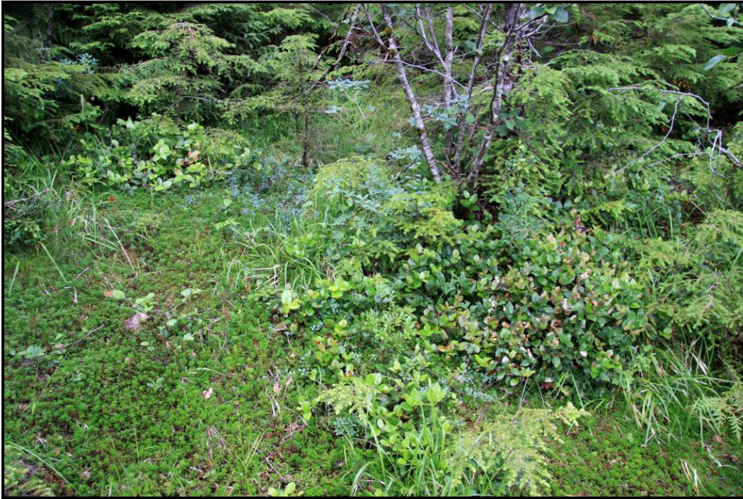
Figure 2-14. Photograph Looking North at the Downstream Face of the Dike, illustrating the type and species of vegetation which have developed over the surface.
