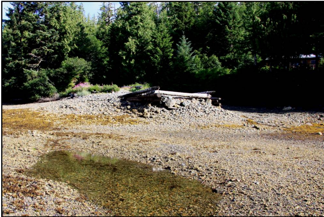
Figure 2-25. Photograph Looking North at the Older and Westernmost Rock Loadout Ramp (Note: Dotson Cabin in the upper right.)
