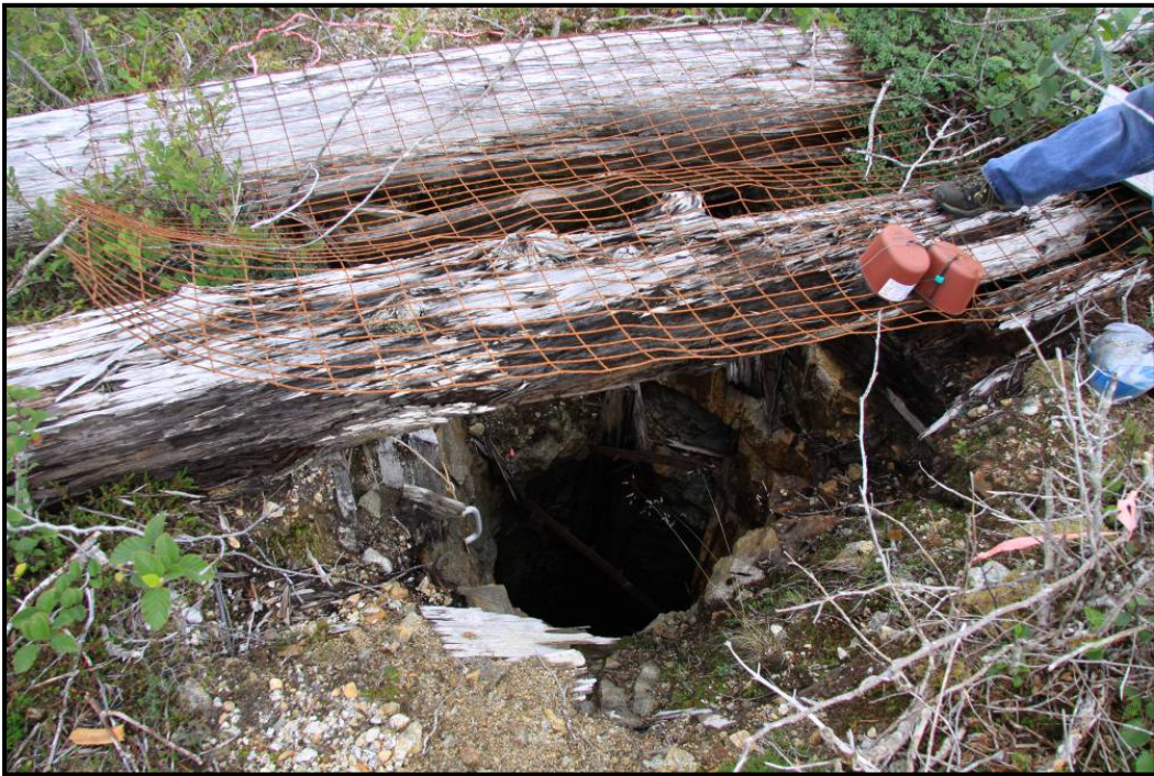
Figure 2-15. Photograph Looking Over the 900-Foot Level Air Shaft (Note the rust colored radon monitoring canisters on the right.)
