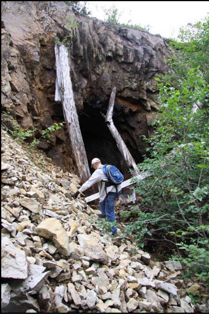
Figure 2-11. Photograph Looking Southwest at the 900-Foot Level Portal
