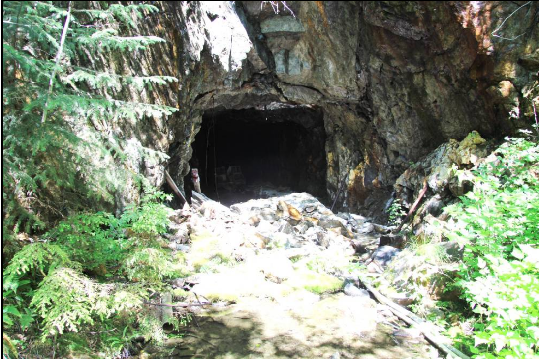
Figure 2-21. Photograph of 300-Foot Level Portal
