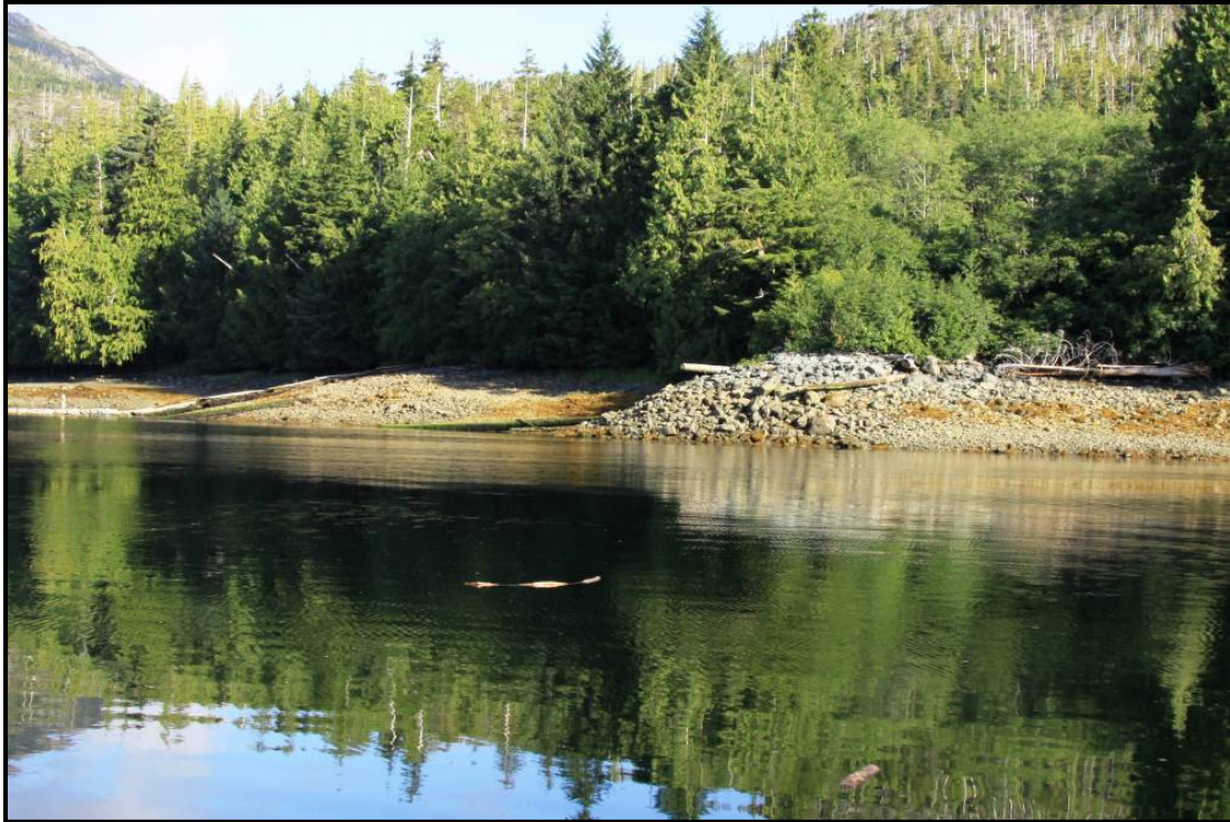
Figure 2-24. Photograph Looking Northwest at the Two Rock Loadout Ramps. (The Ore Staging Area is just beyond the docks.)
