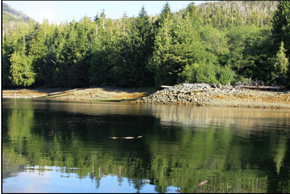
Figure 4-33. Photo looking northwest at the two rock loadout ramps (The Ore Staging Area is just beyond the docks).
