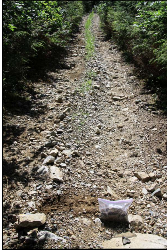
Figure 4-35. Photo looking northwest up the 900-Foot Level haul road, illustrating how dense vegetation has narrowed the road widths
