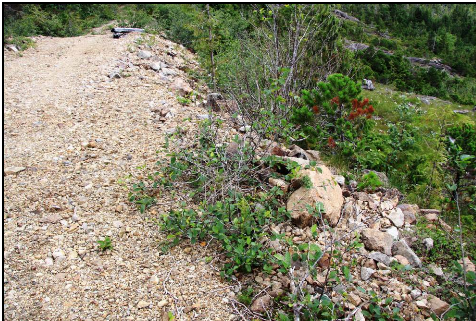
Figure 4-26. Photo looking northeast along the south side of Mine Rock Pile III between the 700- and 900-Foot Levels (This photo shows the typical thickness and material size of all of the mine rock used to construct roads between these two levels of the mine).
