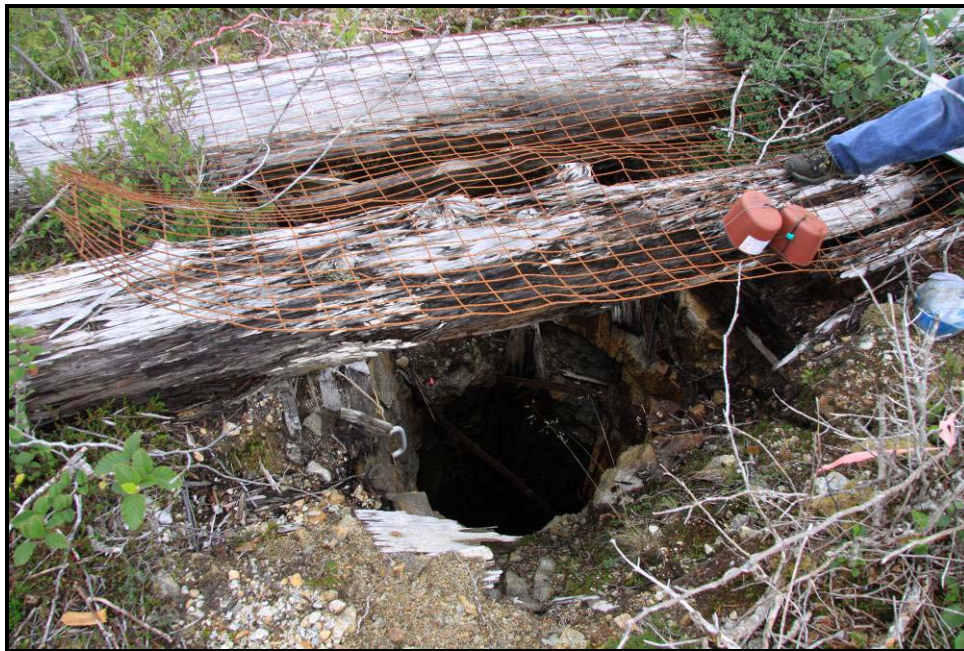
Figure 4-22. Photo looking over the 900-Foot Level air shaft (Note the rust-colored radon-monitoring canisters on the right).
