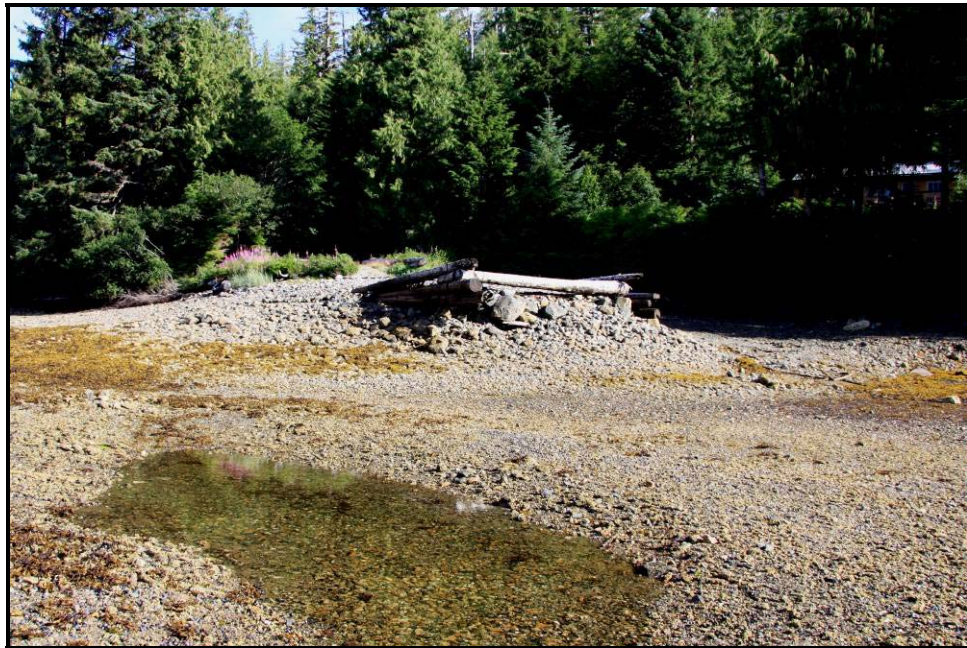
Figure 4-32. Photo looking north at the older and westernmost rock loadout ramp (Note: Dotson Cabin in the upper right).
