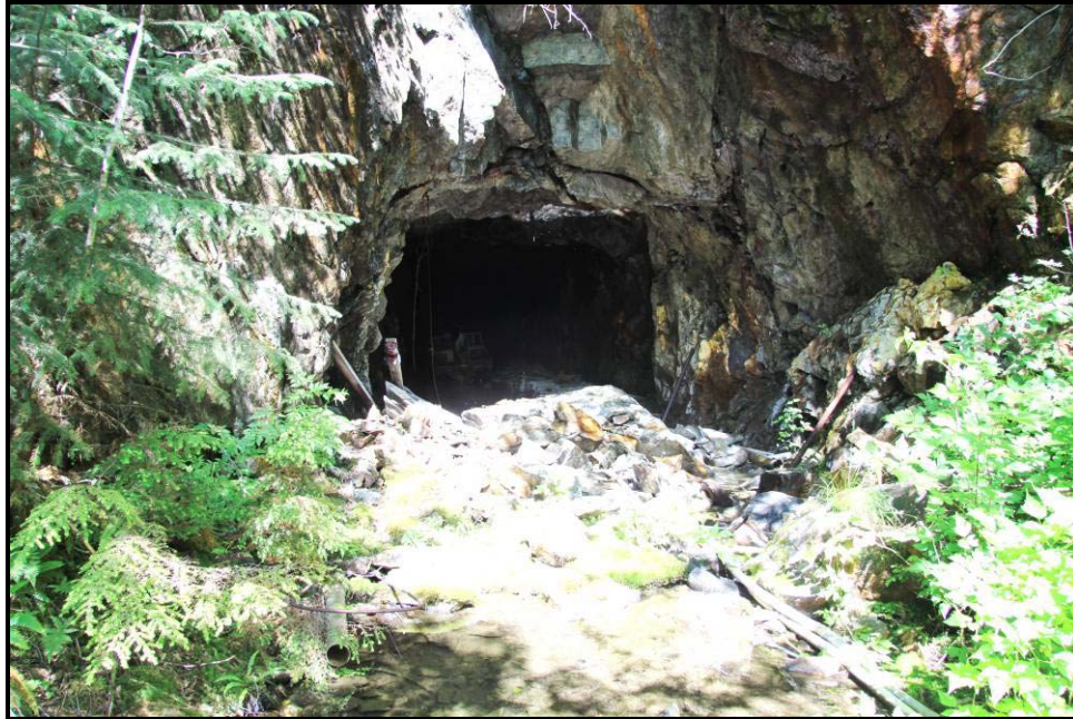
Figure 4-29. Photo of 300-Foot Level portal
