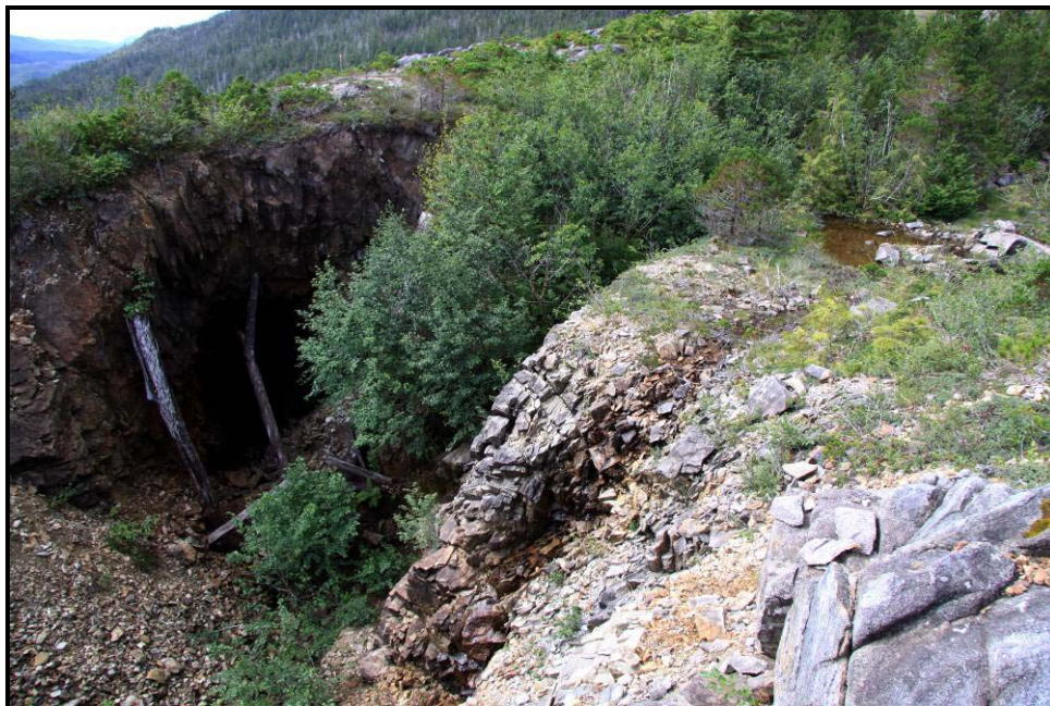
Figure 4-18. Photo looking southwest down into the Open Pit and 900-Foot Level portal showing the point at which surface runoff from the north and west (seen on the right side) enters the pit
