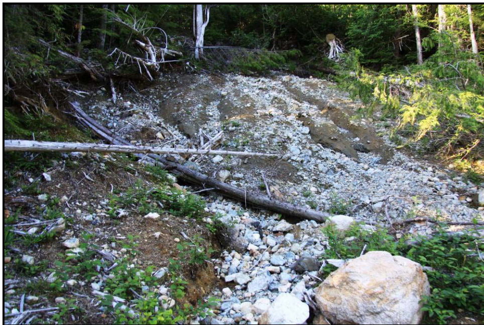
Figure 4-40. Photo looking uphill at the head scarp of the east landslide, illustrating the shallow nature of the slide (Note: The south edge of the 300-Foot Level haul road is located at the upper edge of the head scarp).
