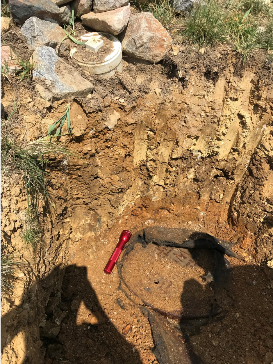
Photo 3. Top of McLaren Adit drain system access manhole (fabric removed).
