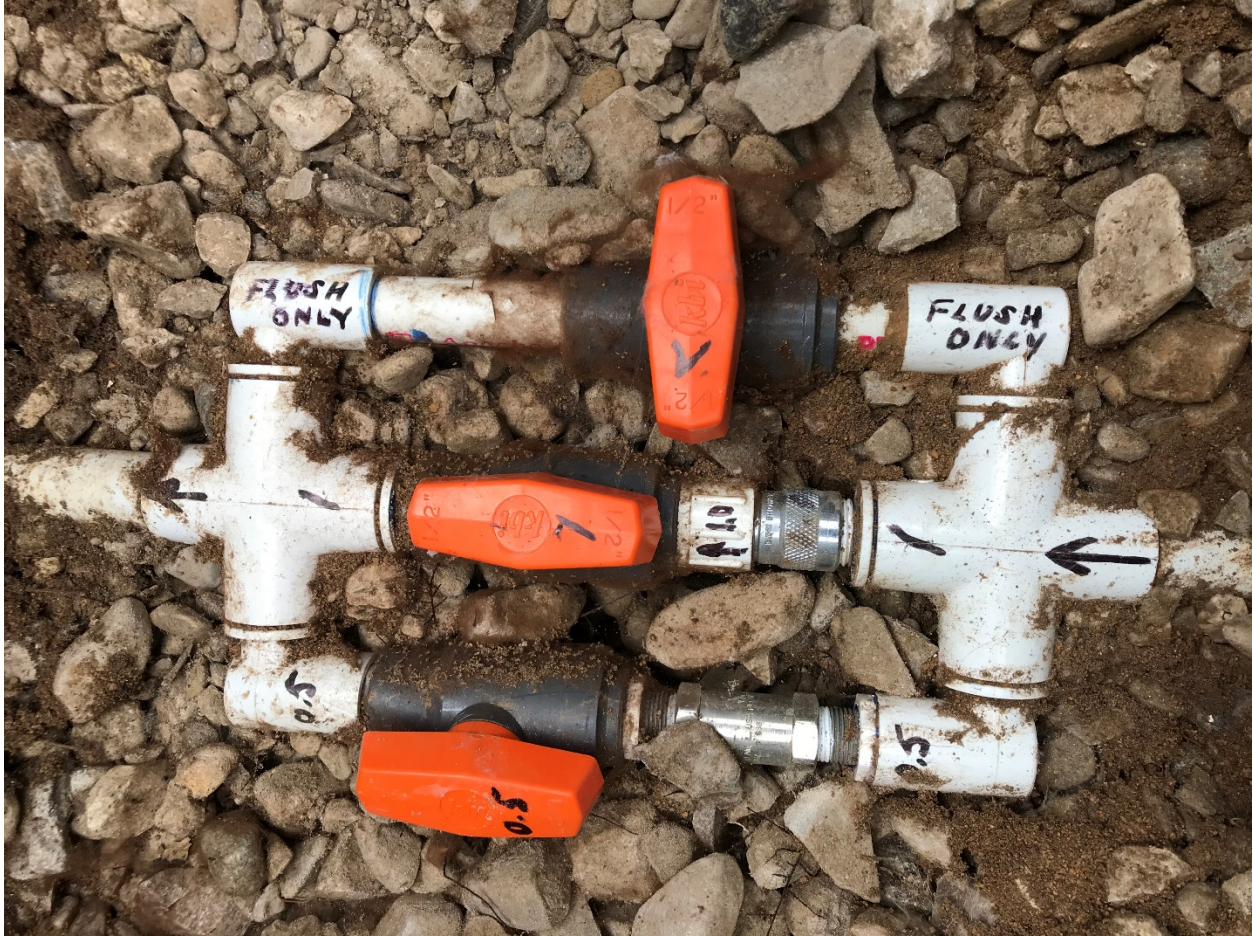
Close up inside western valve box
