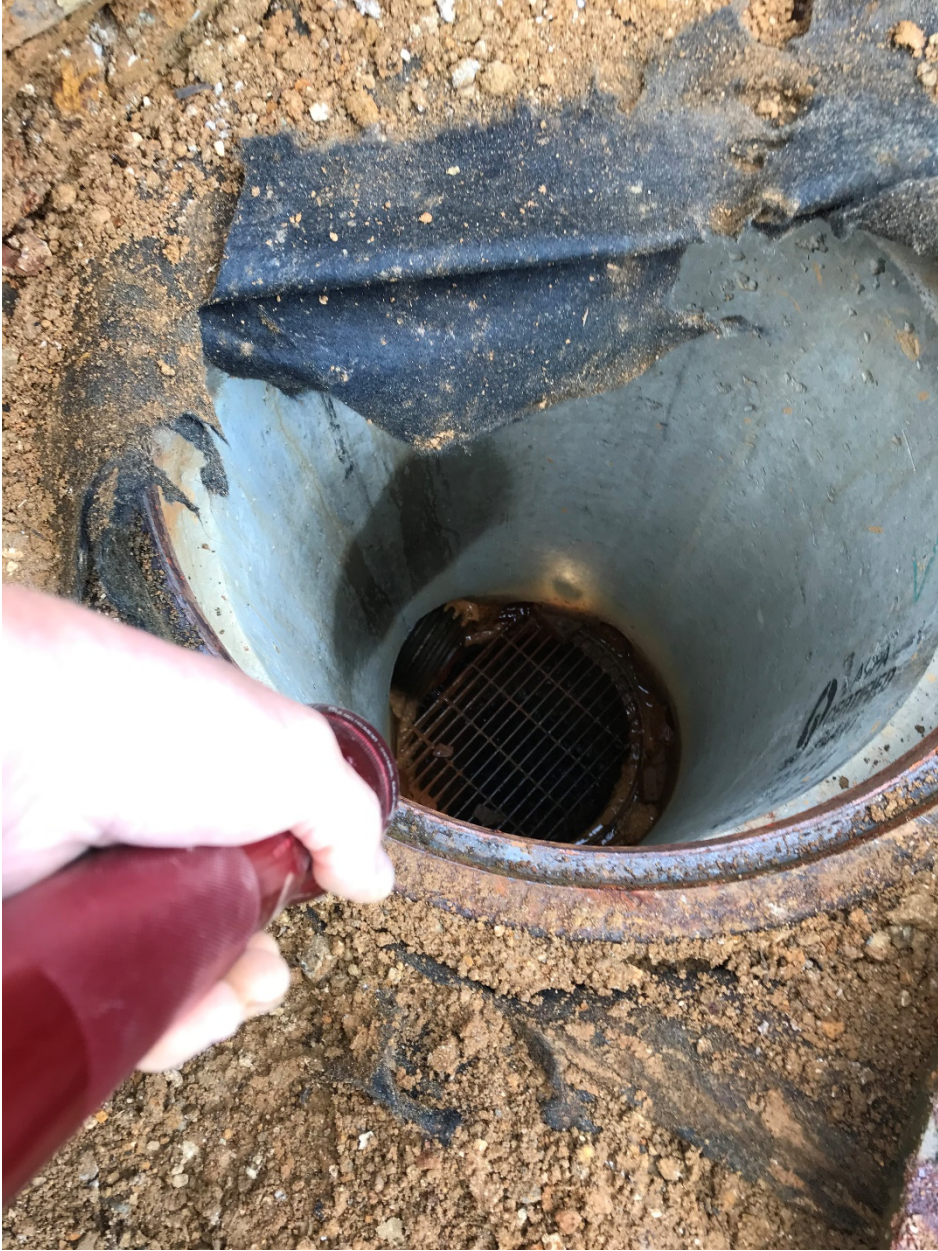
Photo 4. Interior of drain system vault with manhole cover removed.
