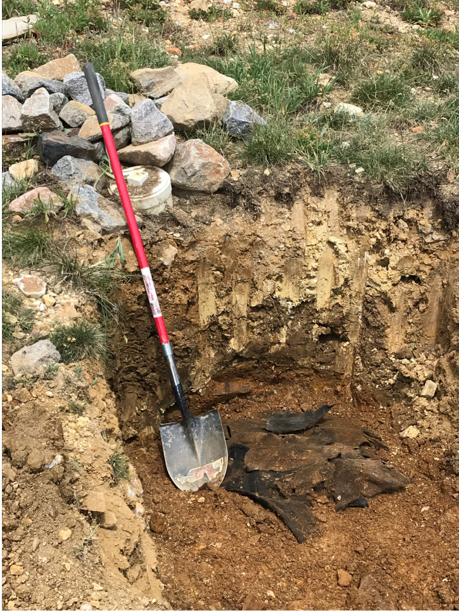
Photo 2. Top of McLaren Adit drain system access manhole (covered with fabric).
