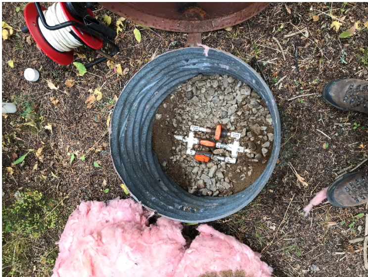
Inside of western valve box
