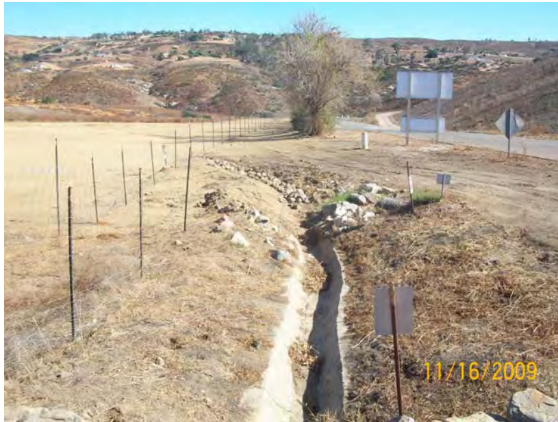
Photograph A-3. Overview of channelized surface water drainage from Allied Waste property onto Forest Service property (left side of photograph). Fenceline is approximate property boundary.
