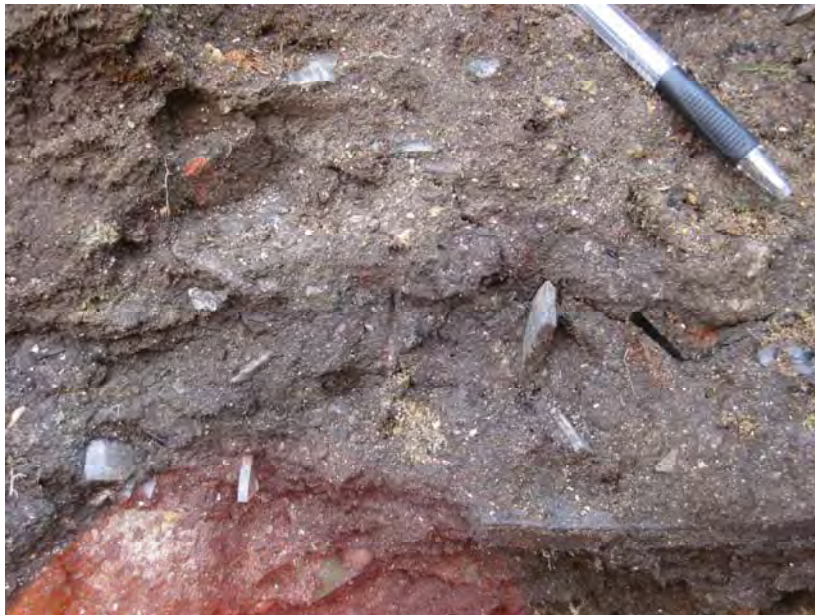
Photograph A-16. Closeup of burn ash and debris exposed in large scour in drainage along northeast edge of site.
