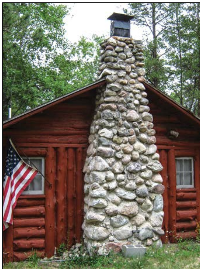
Figure 11—The fieldstone chimney extends well above the roof of this 1957 recreation residence at the Rollways tract of the Huron-Manistee National Forest in the Eastern Region. Smoke rises properly through this chimney that meets code requirements. A metal spark arrester prevents the escape of burning material that could ignite a forest fire.
