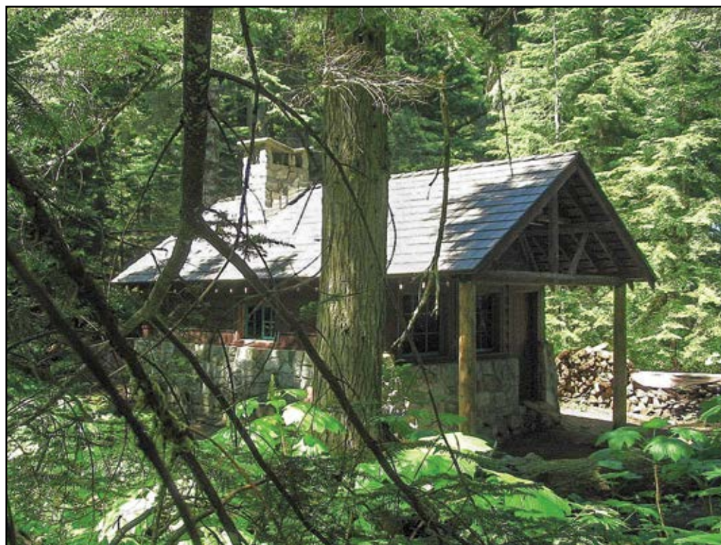
Figure 8—A tree fell during a storm and destroyed most of the original roof of this 1950 recreation residence at the Denny Creek tract of the Mt. Baker-Snoqualmie National Forest in the Pacific Northwest Region. The new roof structure and materials match the appearance of the historic roof, although the structure was strengthened to meet code requirements for snow loading.
