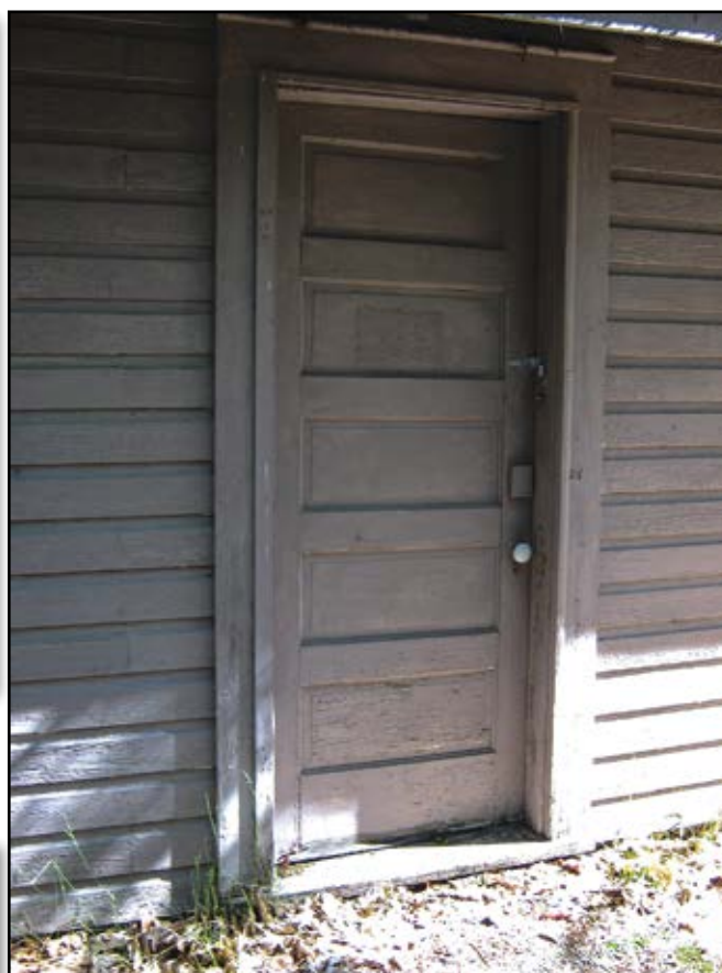
Figure 18—This rail and stile door is original to a mid-20th century recreation residence at the High Rollways tract of the Huron-Manistee National Forest in the Eastern Region.
