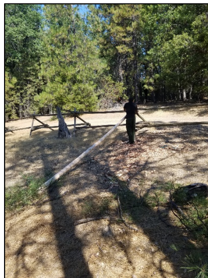
Howard Meadow campground falling trees and peeling them to fix the buck and rail fence
