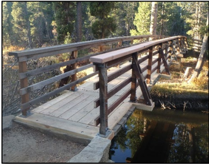
Repaired Chappell Bridge heading into Desolation Wilderness
