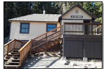
Van Vleck Bunkhouse and Deck Repainted
