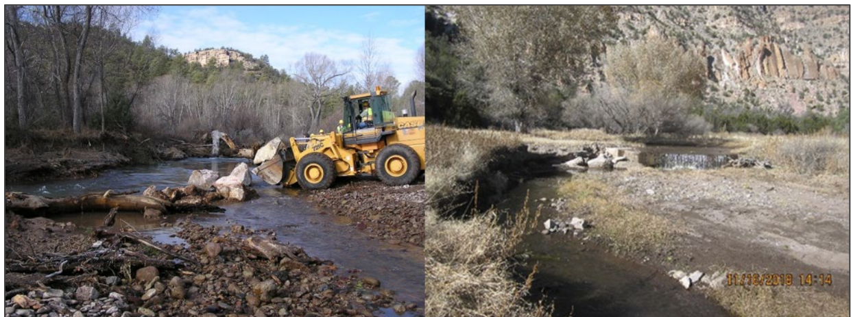
Figure 85. Temporary berm to divert water from project area. Downcutting on stream below a low water crossing.
