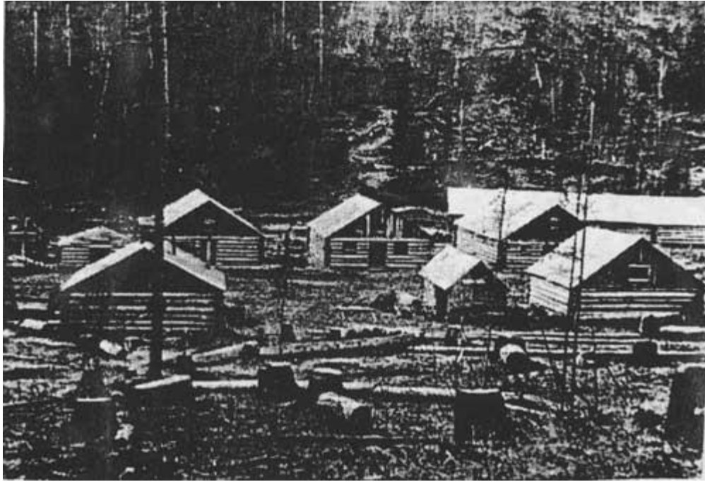
Figure 112. Logging camp known as camp 3, Fortine, Montana (photo courtesy of Henry Elwood).
