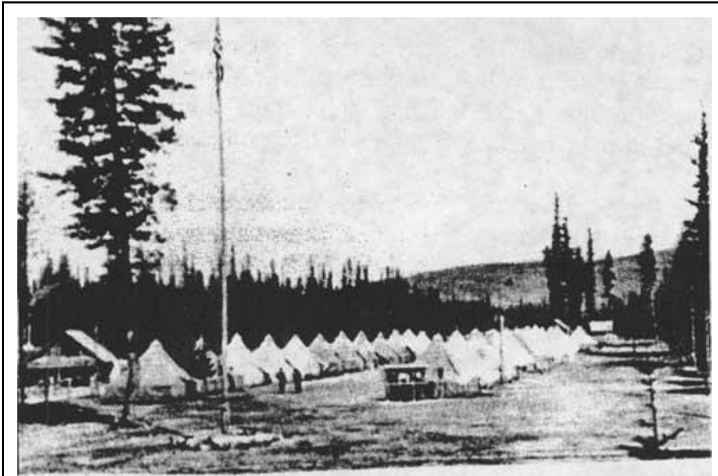
Figure 133. Elk Park (Bridgehead) CCC Camp (F-48), 1935 (courtesy of Flathead National Forest, Kalispell).
