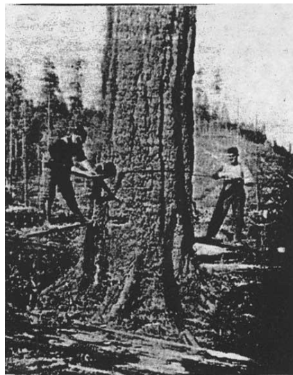
Figure 100. Sawyers felling a Douglas-fir with a cross-cut saw, standing on springboards (Brown 1934:11).
