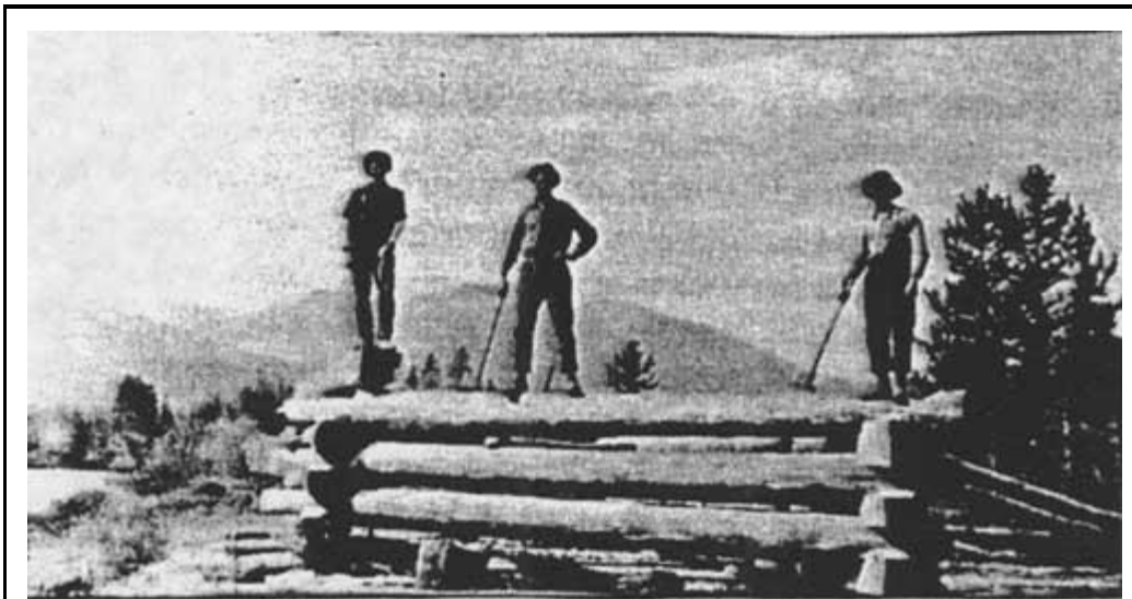
Figure 46. Fitting the abutment timbers on the Big Prairie bridge over the South Fork, 1922 (courtesy of Flathead National Forest, Kalispell).
