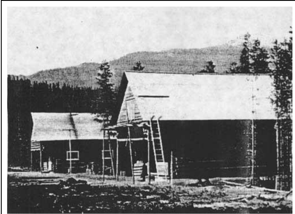
Figure 32. Garage/blacksmith shop under construction at Spotted Bear Ranger Station, 1925. Master log carpenters Vic Holmlund and Everett Hart probably helped build these buildings, which are currently known as the fire cache and the old office (photo by Everett Hart, courtesy of Flathead National Forest, Kalispell).
