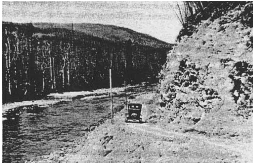
Figure 51. South Fork road near Upper Twin Creek, 1926 (courtesy of Flathead National Forest, Kalispell).
