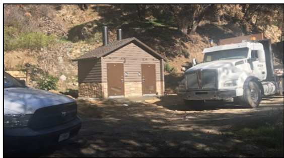
Robert's Camp, Chantry Flat Picnic Area, with a new modern, precast concrete lined toilet
