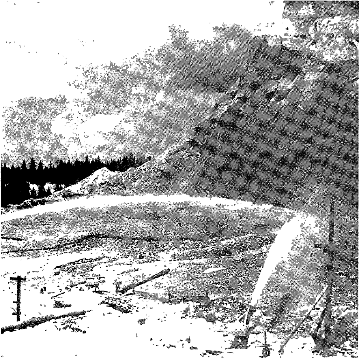
Hydraulic Mining. Omega Mine, c 1920
