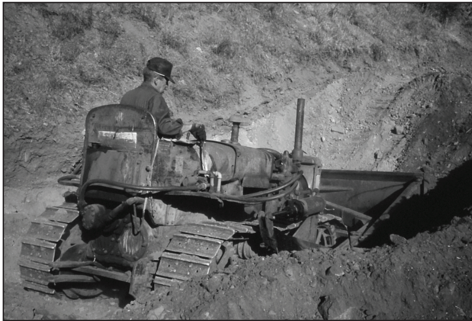
Francie Wallace digging a grave for the dozer, 1975 — USFS
