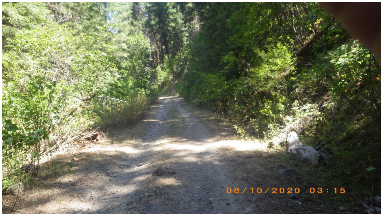
Figure 5. This project would place large wood and slash in a jackstraw manner after road obliteration authorized by the Big Mosquito project (USDA Forest Service 2015).
