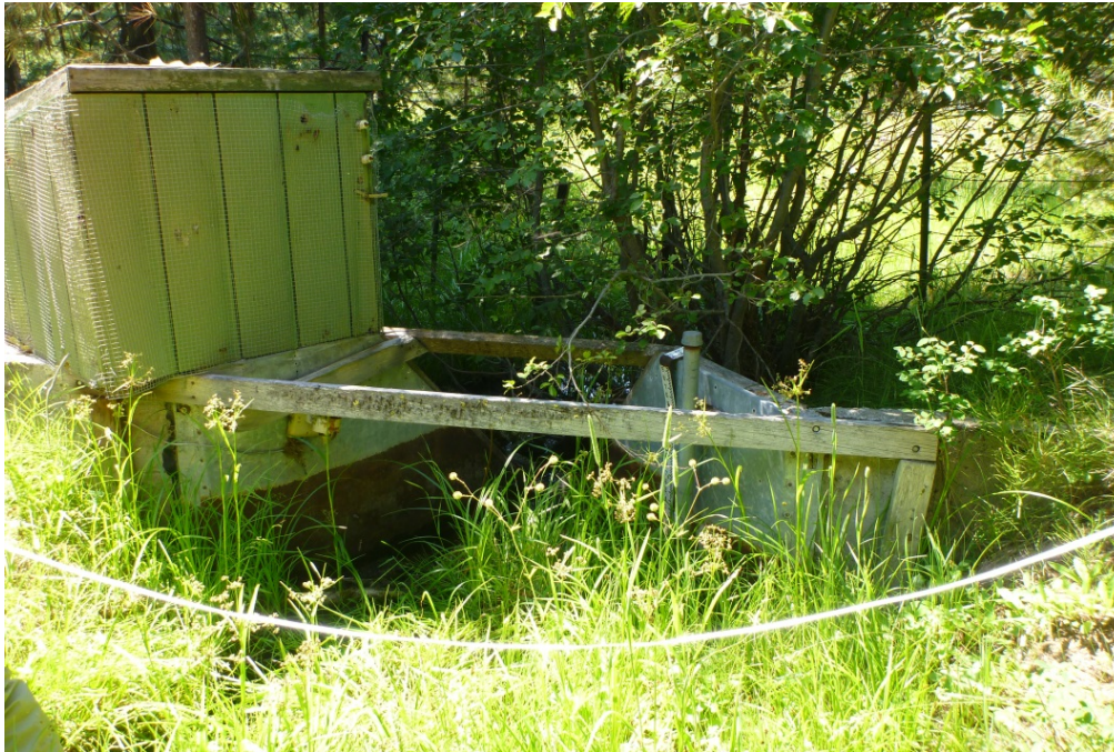
Figure 4. Tinker Creek gauging station and associated wooden structure proposed for removal
