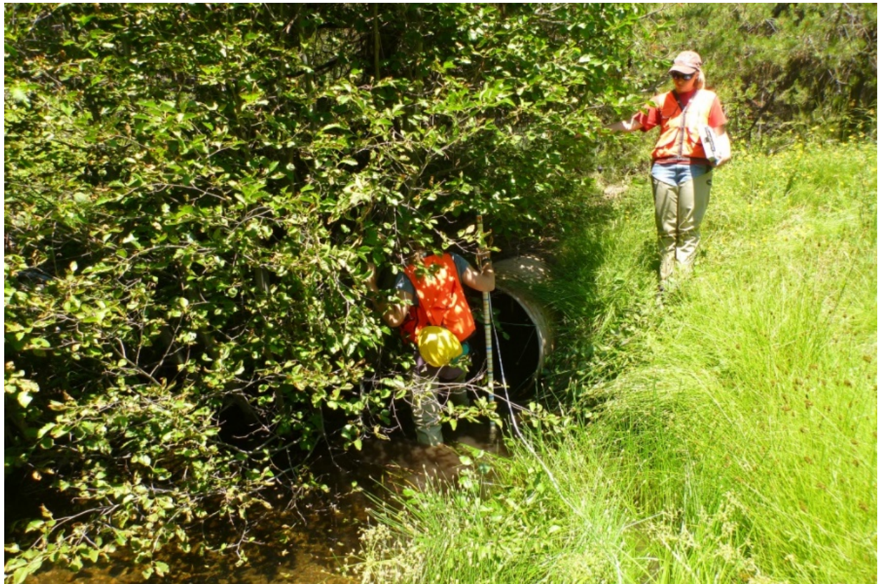
Figure 8. Proposed National Forest System (closed) Road 3620646. Culvert removal looking upstream.
